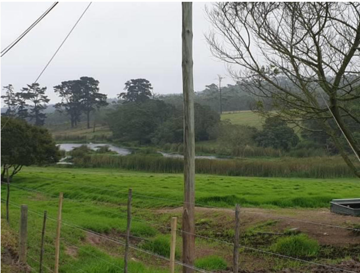
Figure 8: View of the existing irrigation dam
