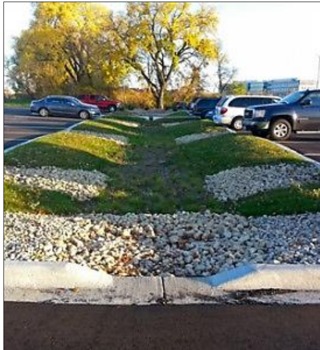
Figure 10: Typical Stormwater Bioretention System at a parking area
