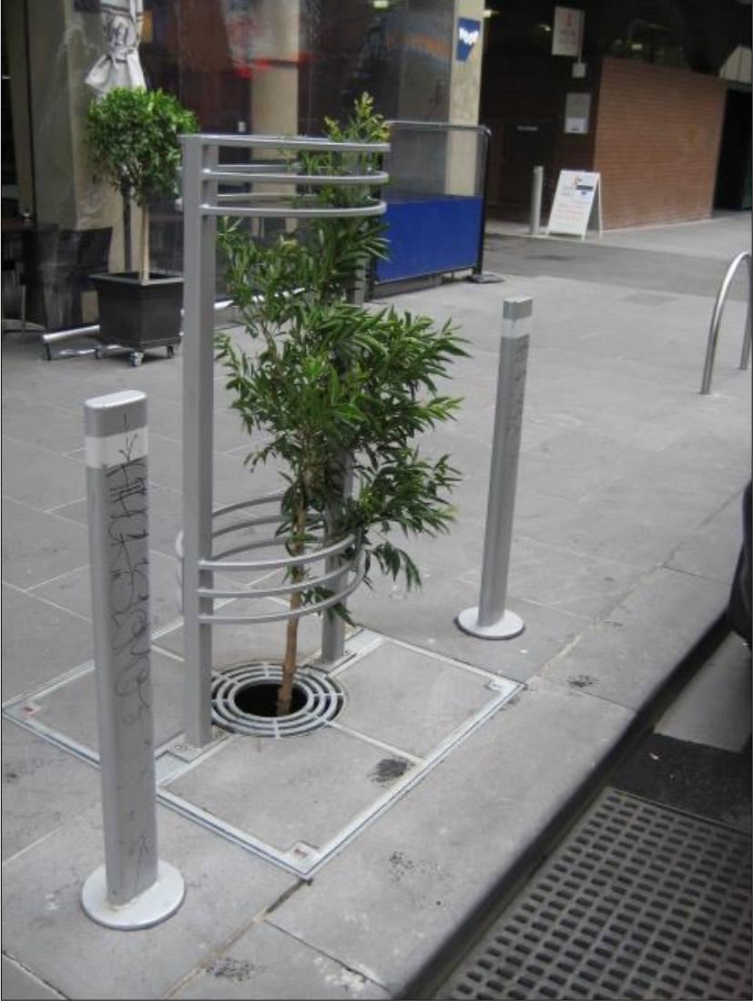
Figure 3 ‘Tree pit’ ( http://urbanwater.melbourne.vic.gov.au/projects/raingardens/little-collins-street-tree-pits/ )
