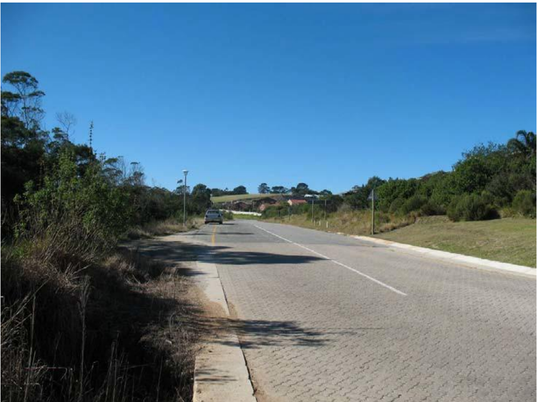
Photo C4: View NW at junction to road to Herold's Bay Ext 1 530m to northern edge of Site
