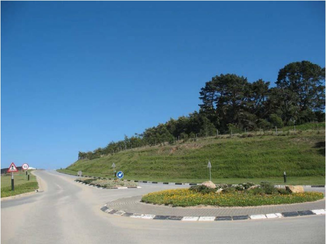
Photo C5a: View West at circle at Breakers View and Oubai Estate
