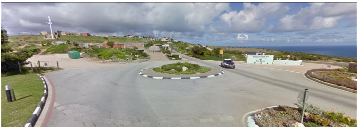
Figure 18: South-eastern view along Oubaa Main Road at the existing traffic circle with the existing and proposed access (gravel road) to the left and the existing accesses to Oubaa Golf Estate and Breakwater Bay Eco Estate in the centre and right respectively. Sight distance is excellent in both the horizontal and vertical alignments.
