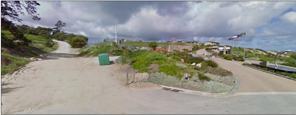
Figure 26: Existing stormwater inlet at the existing traffic circle at the entrance to the proposed development.
