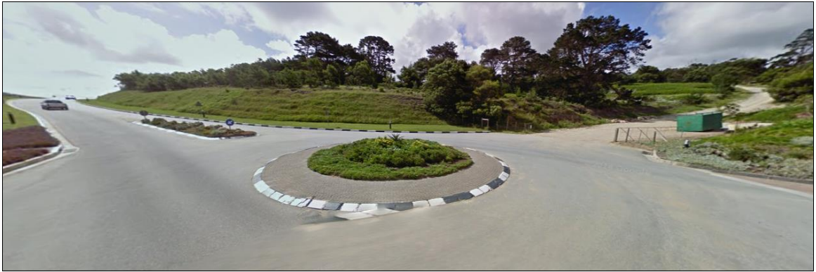
Figure 17: North-western view along Oubaa Main Road at the existing traffic circle with the existing and proposed access (gravel road). Sight distance is excellent in both the horizontal and vertical alignments.
