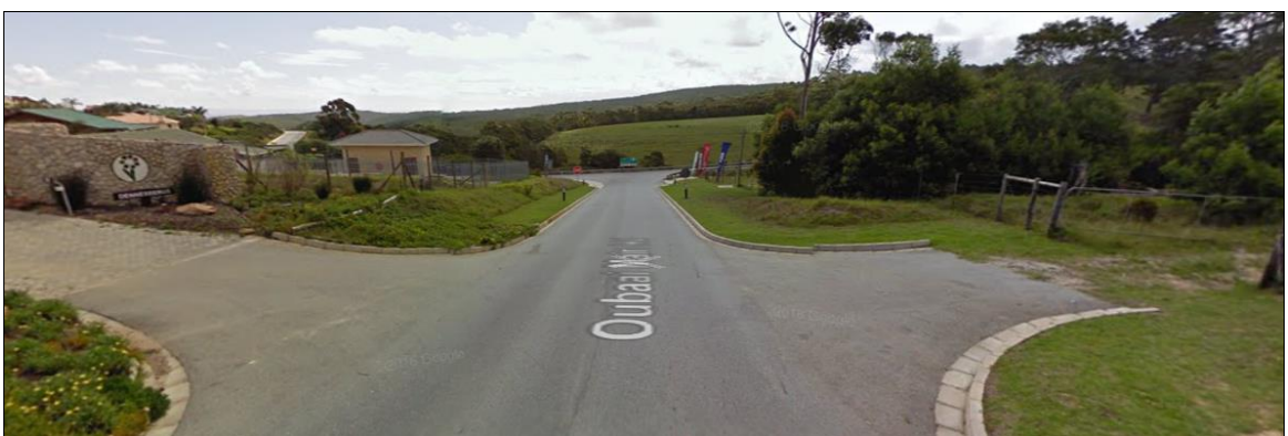
Figure 19: Western view along Oubaa Main Road at the proposed access to the filling station (on the right). Sight distance is excellent in both the horizontal and vertical alignments.
