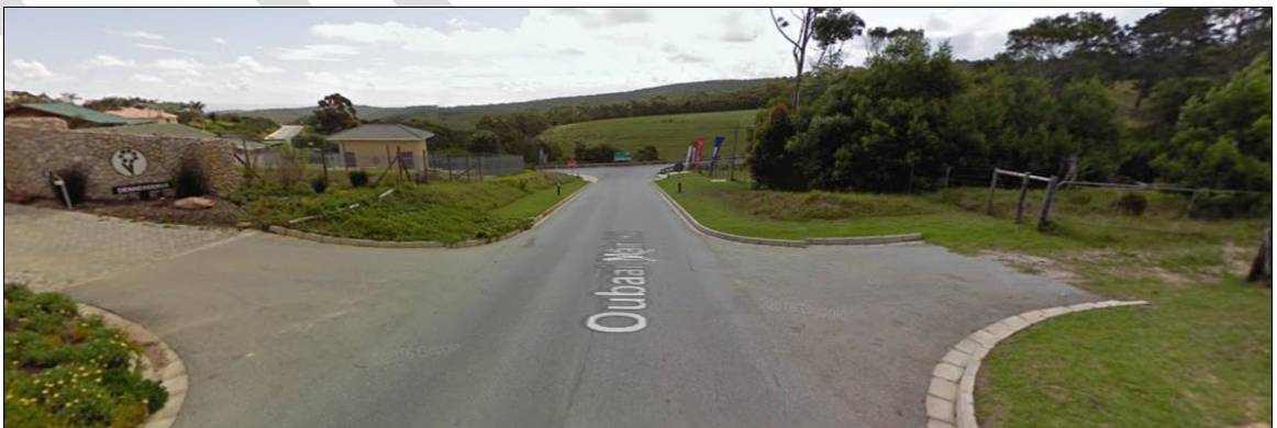
Figure 24: Western view along Oubaa Main Road at the proposed access to the filling station (on the right). Sight distance is excellent in both the horizontal and vertical alignments.
