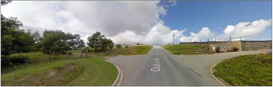
Figure 25: Eastern view along Oubaa Main Road at the proposed access to the filling station (on the left). Sight distance is excellent in both the horizontal and vertical alignments.
