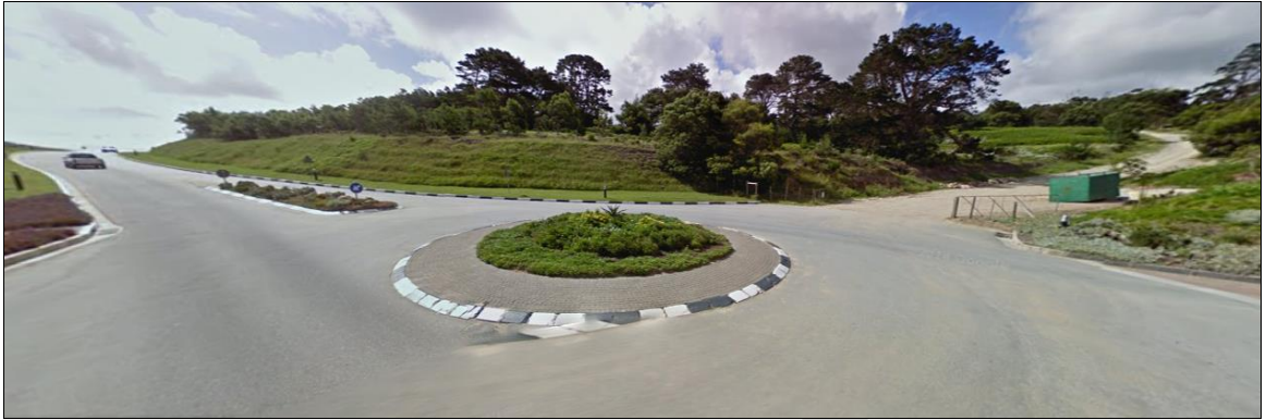
Figure 22: North-western view along Oubaa Main Road at the existing traffic circle with the existing and proposed access (gravel road). Sight distance is excellent in both the horizontal and vertical alignments.
