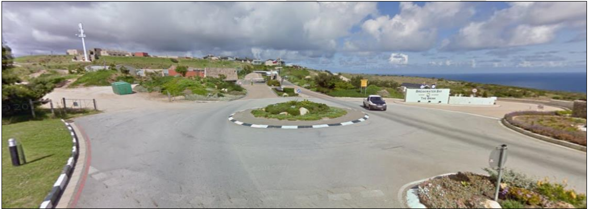
Figure 23: South-eastern view along Oubaa Main Road at the existing traffic circle with the existing and proposed access (gravel road) to the left and the existing accesses to Oubaa Golf Estate and Breakwater Bay Eco Estate in the centre and right respectively. Sight distance is excellent in both the horizontal and vertical alignments.
