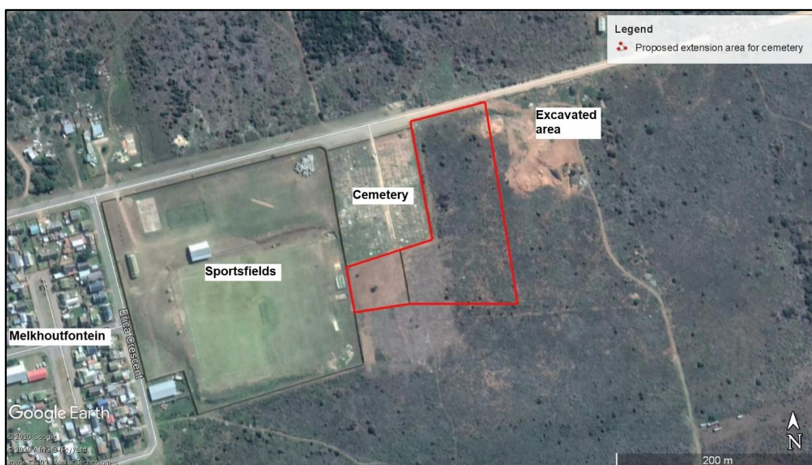
Map 2 Satellite photo showing the position of the study area and footprint of the proposed extension area.
