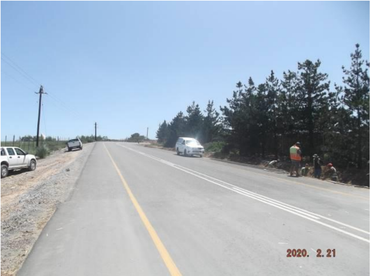
Figure 3: View towards the north along Sorgfontein Road
