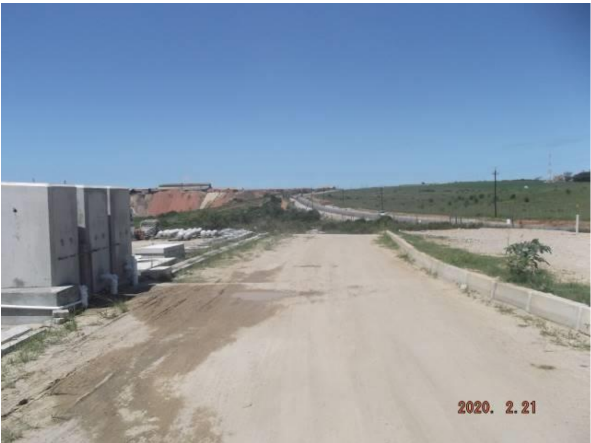
Figure 4: Existing internal access road to the proposed site development area.
