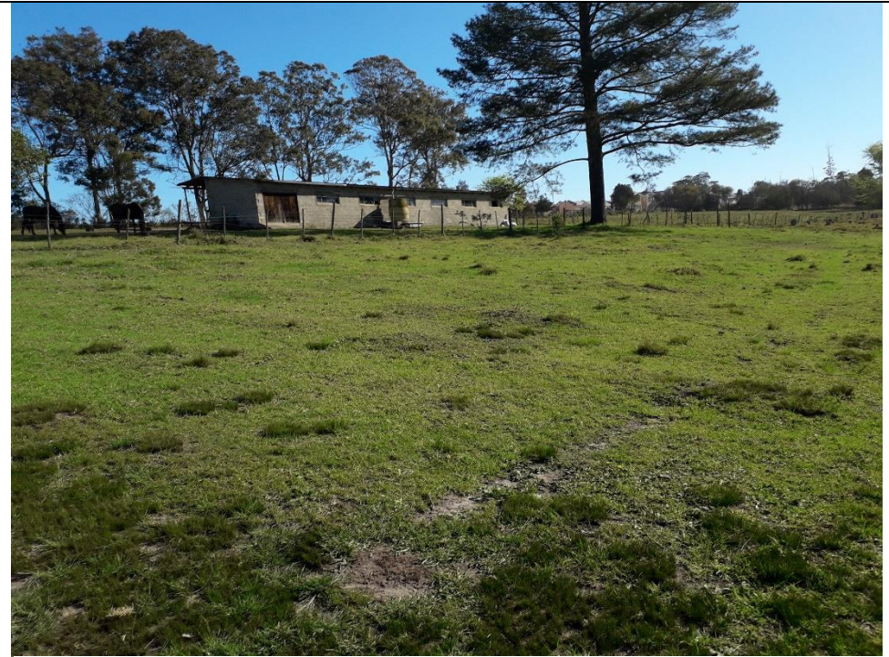
Figure 4: Existing Farm Infrastructure, Looking North West
