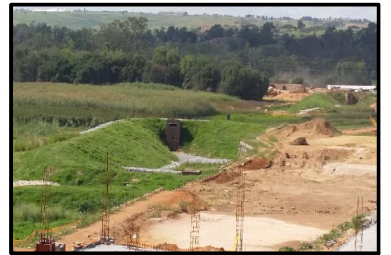
PHOTO OF OUTLET COMPLETED
