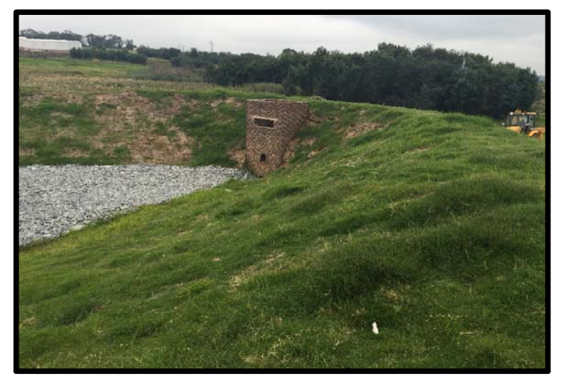
PHOTO OF NEAR-COMPLETED OUTLET
