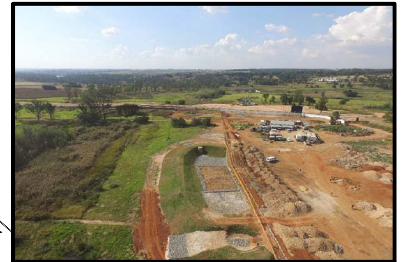
PHOTO OF PONDS ALONG WETLAND
