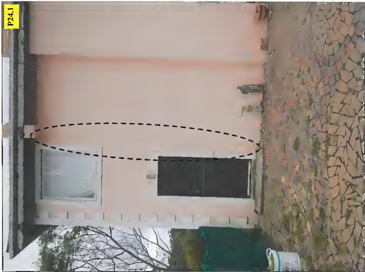
Vertical crack along movement joint, evidently, that runs through the north side of Mr Quintin Olivier's house.
