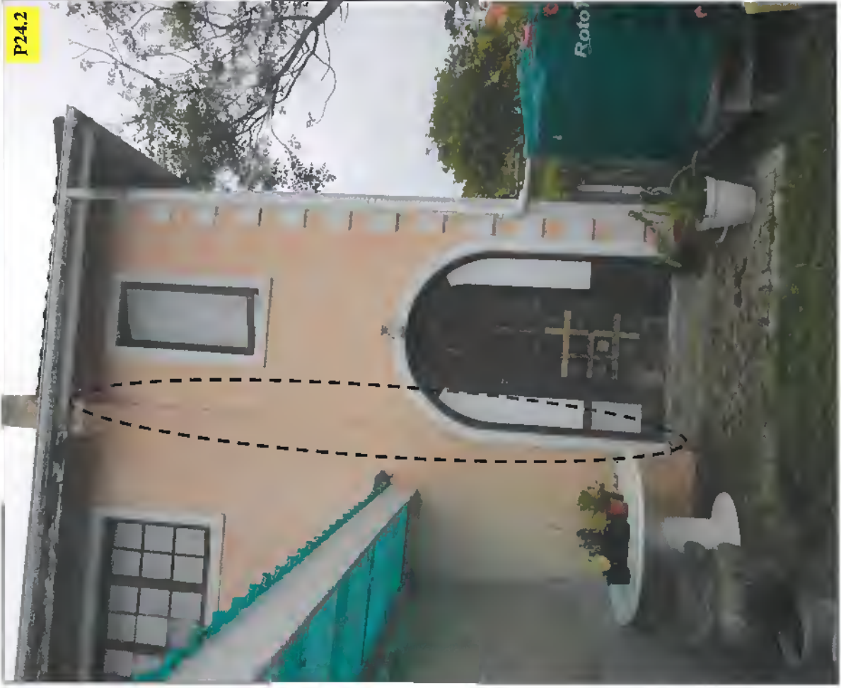
Vertical crack along movement joint, evidently, that runs through the north side of Mr Quintin Olivier's house.
