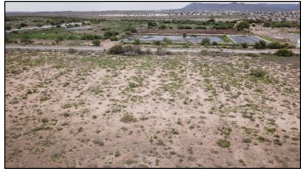
Image 10: Adjacent wastewater treatment works
