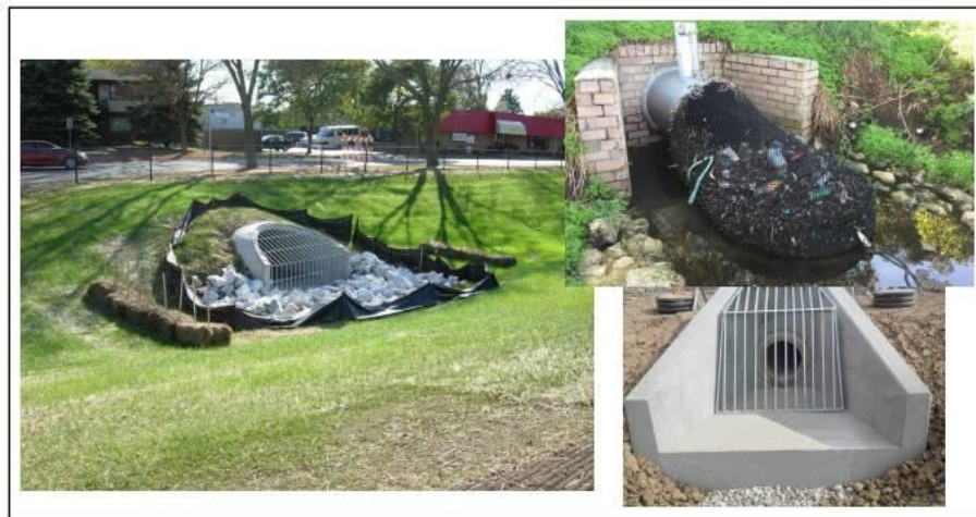
Figure 18: Examples of litter traps - inlet pollution controls
