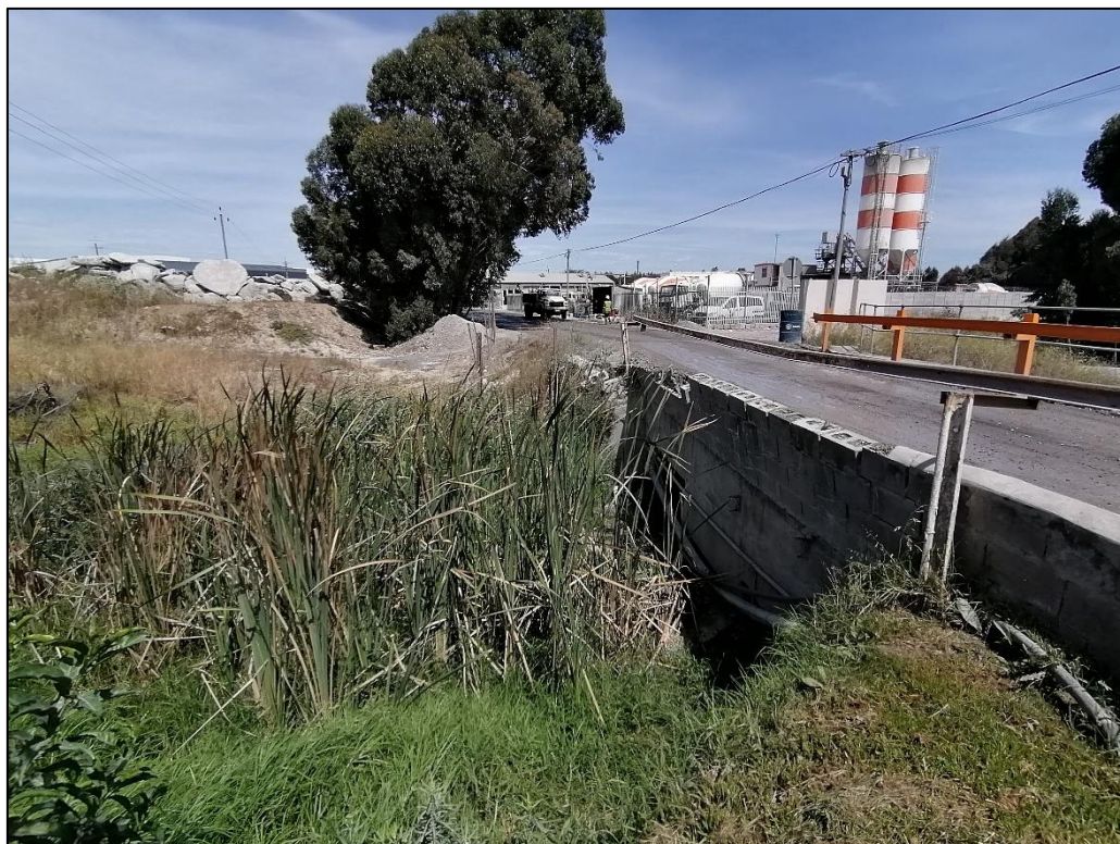
Figure 4: The bridge proposed to be widened
