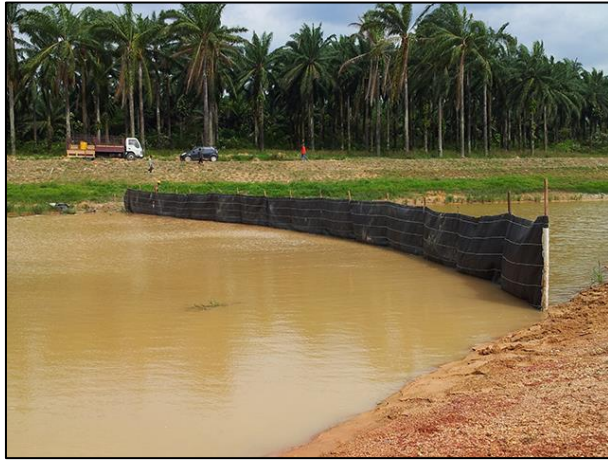
Figure 18: An example of a silt fence placed securely, directly downstream of construction to trap sediment that will then be removed from the riparian habitat
