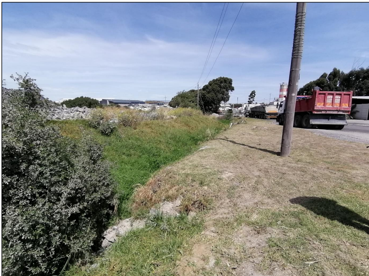
Figure 7: The existing vegetated stormwater drain directing stormwater towards the watercourse near the bridge
