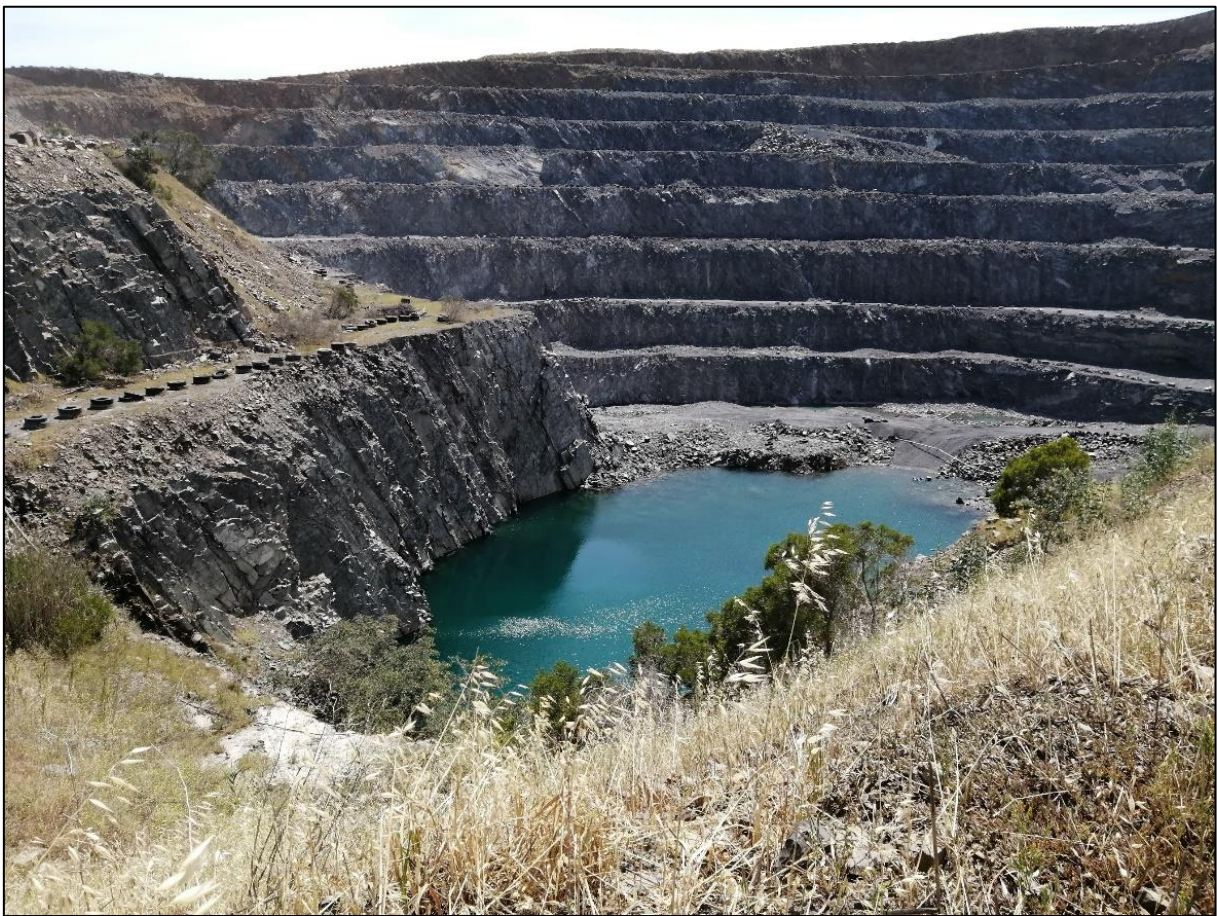
Figure 5: A photo of the quarry temporary water storage pit, during the site visit, following a rainfall event
