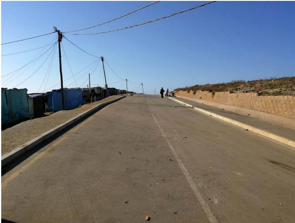
Photo 1: The existing Walvis Street
