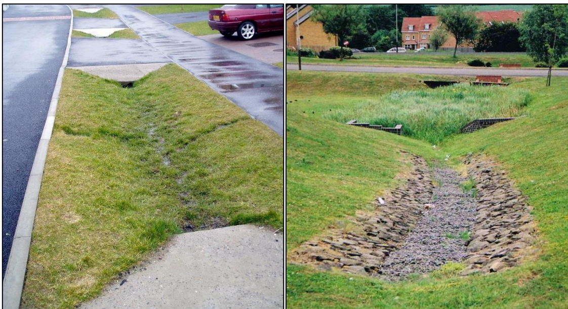
Figure 38: Examples of soft infrastructure incorporated into the stormwater management design (porous channels / swales)
