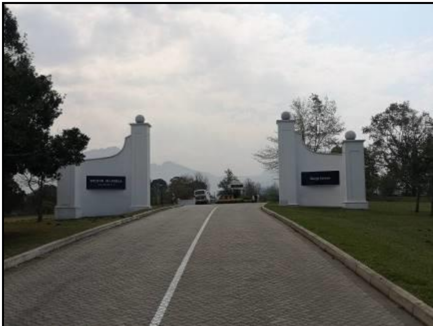
Photograph 3.10: Entrance to NMU Sassveld campus
