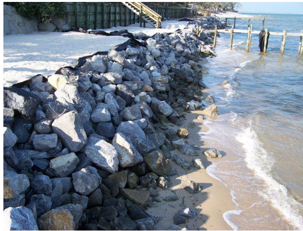
Figure 2. Example of riprap proposed by the GRDM (image supplied by GRDM).
