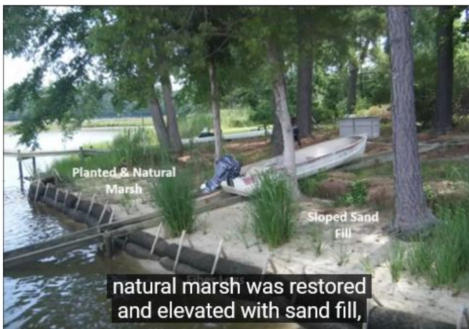
Figure 14. Examples from the Virginia Institute of Marine Science showing the placement of fibre logs and matting (a), followed by infilling with sand and stabilisation with planted vegetation (b).
