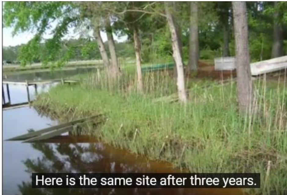
Figure 15. Example of shoreline protection using fibre logs with backfilled sand and planted marsh (Virginia Institute of Marine Science).
