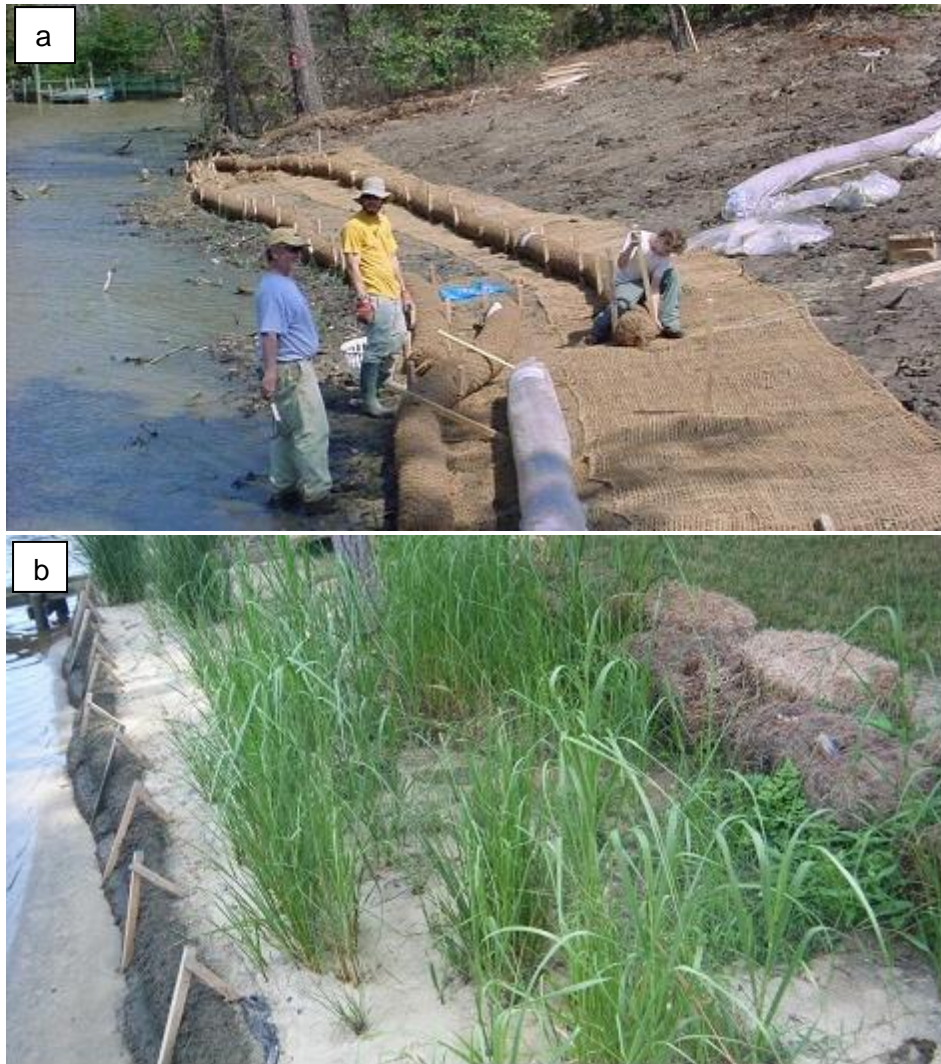
Figure 14. Examples from the Virginia Institute of Marine Science showing the placement of fibre logs and matting (a), followed by infilling with sand and stabilisation with planted vegetation (b).
