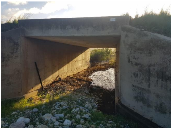
Image 77: Major Culvert C10615 flow path.
