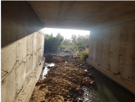
Image 79: Major Culvert C10615 flow path.
