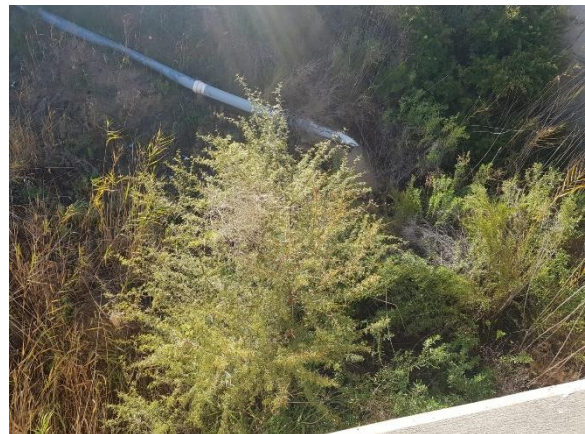
Image 113: Piping infrastructure within the watercourse.
