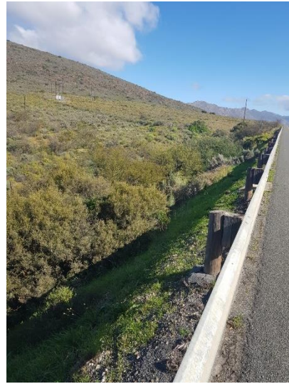
Image 132: Adjacent topography showing a steep gradient.
