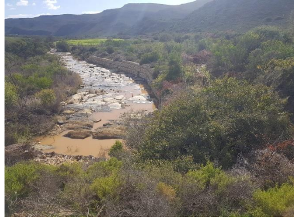
Image 127: Eastern flow path and adjacent vegetation.
