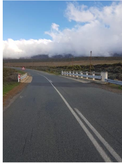
Image 2: Koo River Bridge.
