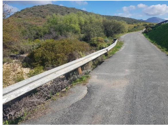
Image 121: Side access road.
