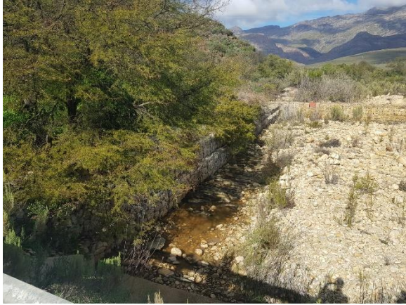
Image 126: Adjacent riverine vegetation and gabions.
