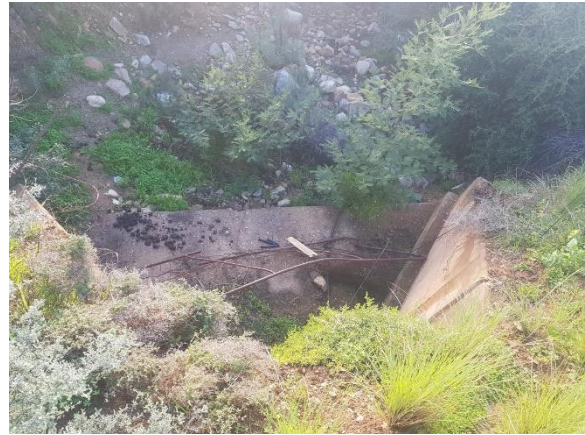
Image 69: Metal gate within flow path.
