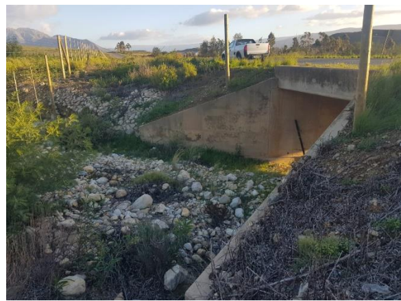
Image 82: Major Culvert C10615 flow path and adjacent topography.
