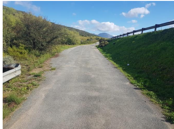
Image 123: Side access road.
