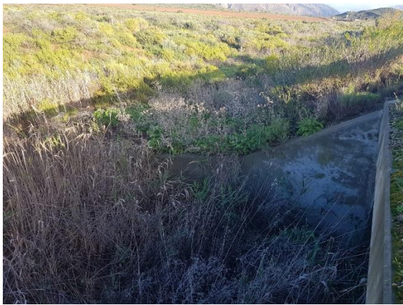
Image 93: Topography adjacent to the Culvert.
