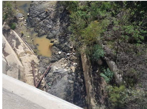
Image 149: Concrete pillar within flow path.
