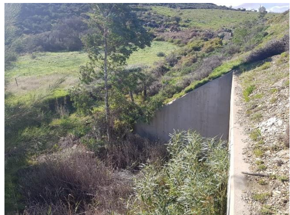
Image 140: Adjacent topography showing a steep gradient.
