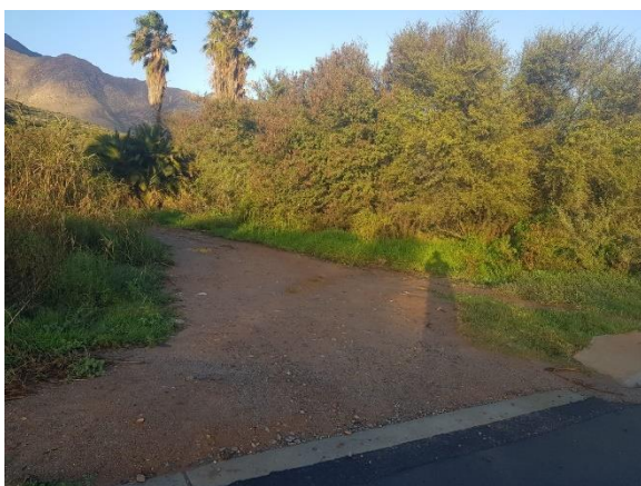
Image 66: Side access road adjacent to bridge.
