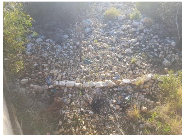
Image 78: Major Culvert C10615 flow path well sorted.
