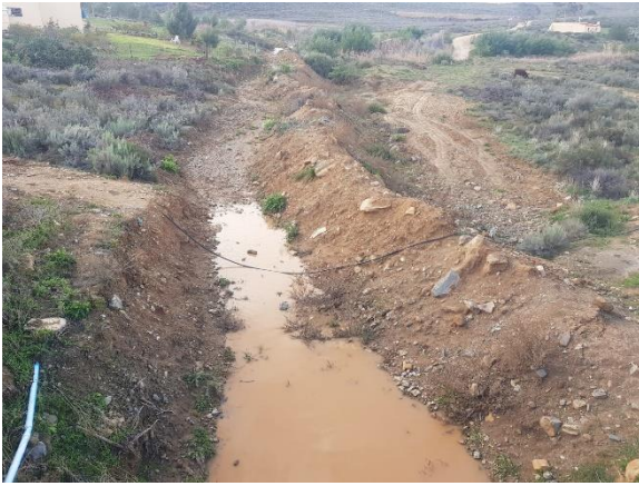
Image 28: Watercourse with disturbed adjacent areas.
