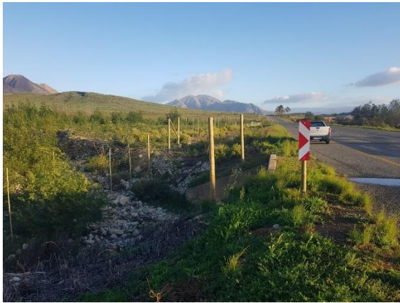
Image 75: Major Culvert C10615 and fence line.
