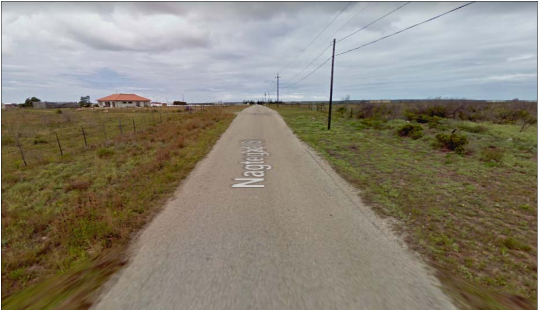
Figure 8: Southern view along Nagtegaal Street at the access point. Sight distance is excellent in both the horizontal and vertical alignments.
