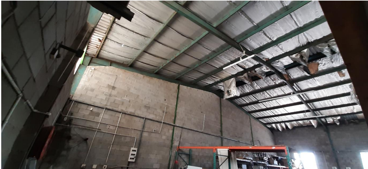
Figure 21: Disrepair of the interior roof on eastern side of warehouse.
