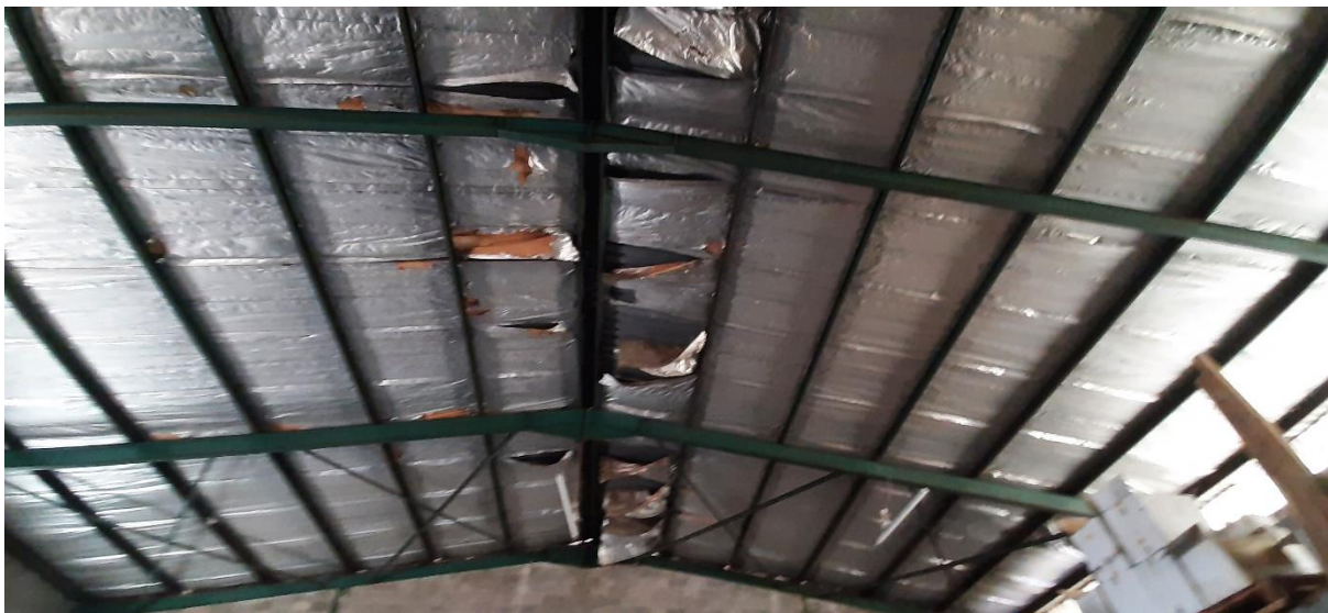
Figure 20: Disrepair of interior roof of the central portion of the warehouse.
