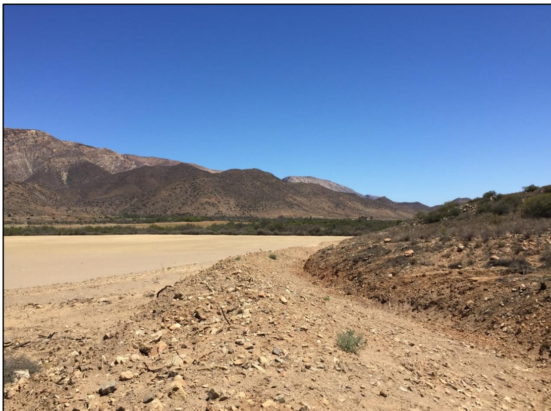
Photo 8 Stormwater cut-off trench above western new land.
