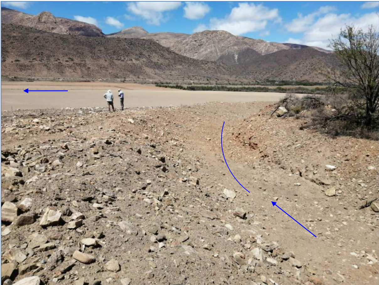
Figure 35: The lower reach of the stream channel has been modified and a cut-off berm diverts the flow around the northern edge of the lands
