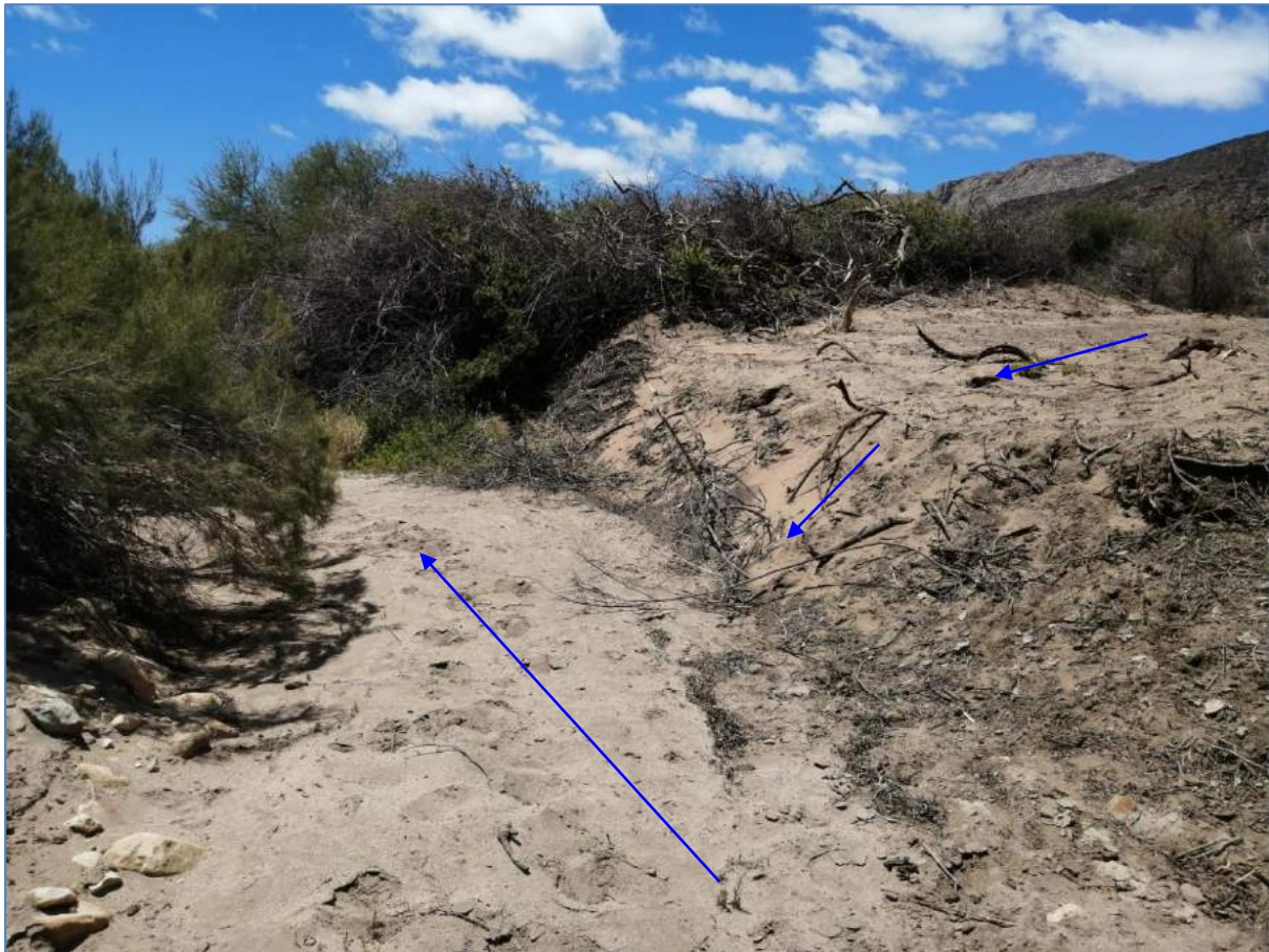
Figure 40: The excavated channel directing surface flow and sediment into the channel of the Cordiers River
