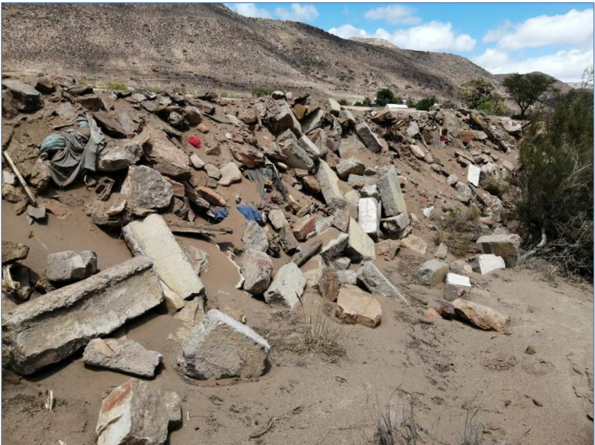
Figure 27: Infilling of the channel with rubble in order to divert flow from the lands
