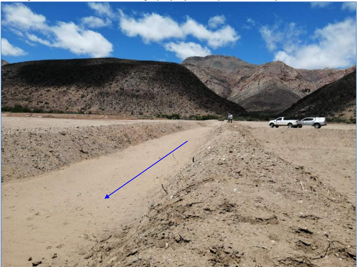
Figure 39: The excavated channel directing any surface flow directly into the channel of the Cordiers River from the road
