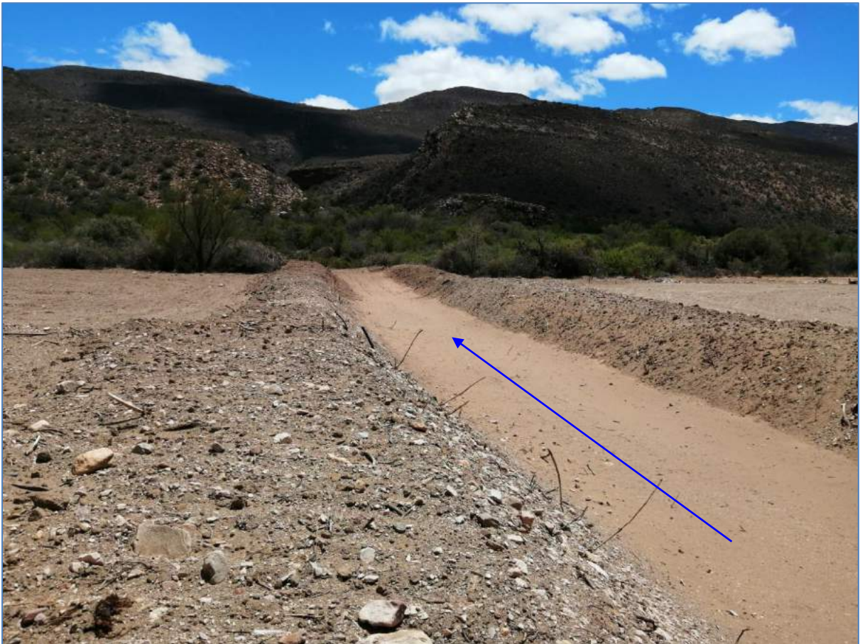
Figure 38: The excavated channel directing any surface flow directly into the channel of the Cordiers River
