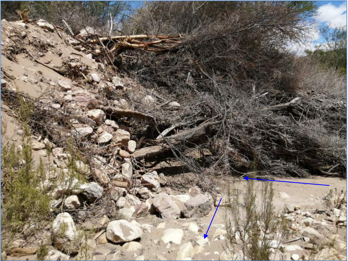
Figure 28: Infilling along the bank of the Cordiers River to protect lands from natural channel migration
