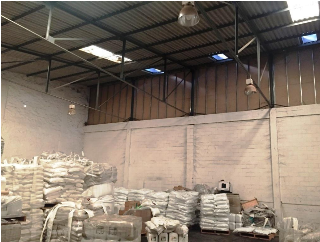
Photo 3: Internal Warehouse A – dividing wall
