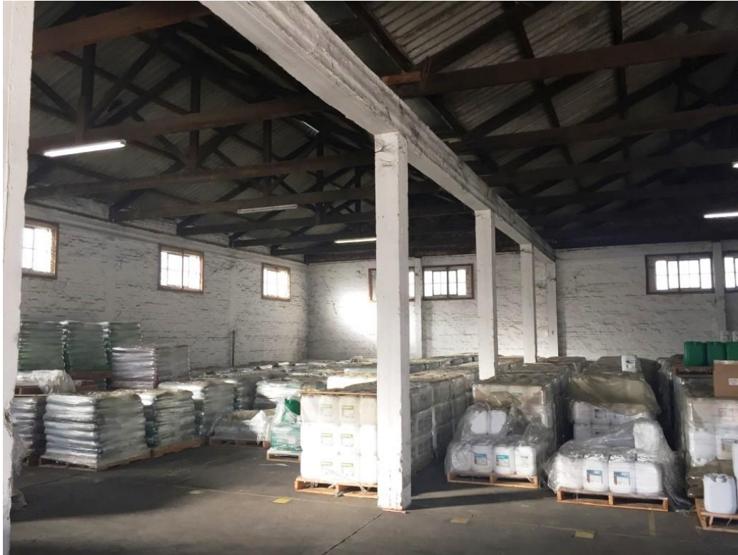
Photo 4: Internal Warehouse B – RC Frame
