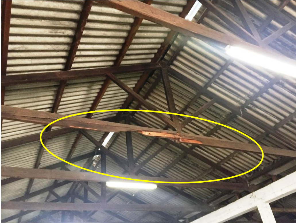
Photo 1: Damaged timber truss in Warehouse B
