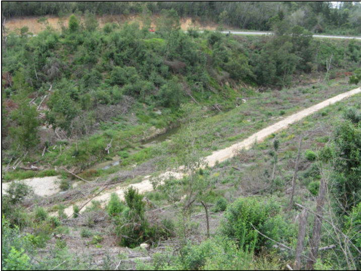
PHOTO 9: The minor stream which has become polluted by municipal sewerage discharge has been negatively impacted by the nutrient-rich effluent.
