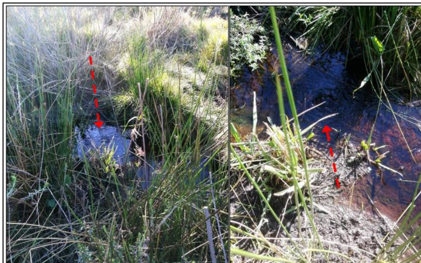
Figure 29: Photographs showing the source of water inputs from a leaking water pipeline
