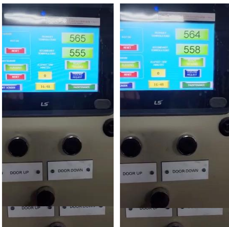
Figure 6: Images above showing the secondary chamber temperature rising progressively from 555 °C to 576 °C, while the first chamber temperature is stable. Figure 7 shows the emissions at this point.
