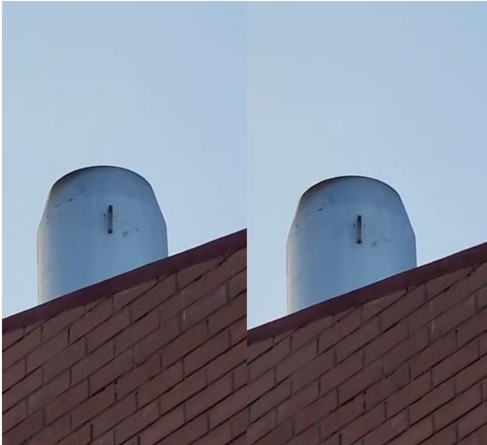
Figure 7: No visible emissions are released from the chimney stacks at the point of a primary chamber temperature of 565 °C and the secondary chamber temperature of 576 °C. The process of cremation has not started at this point.
