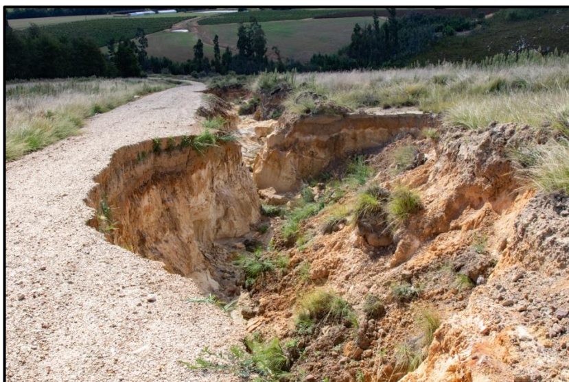
Figure 21. Sections of the access road were almost completely washed away.
