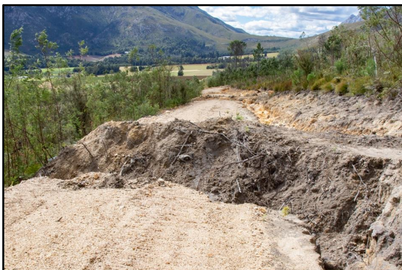
Figure 18. Dongas were formed across the access road by the stormwater runoff.
