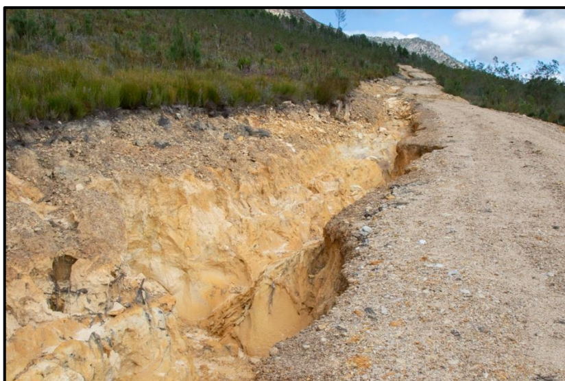
Figure 19. A deep donga down to bedrock formed on the upper side of the access road.
