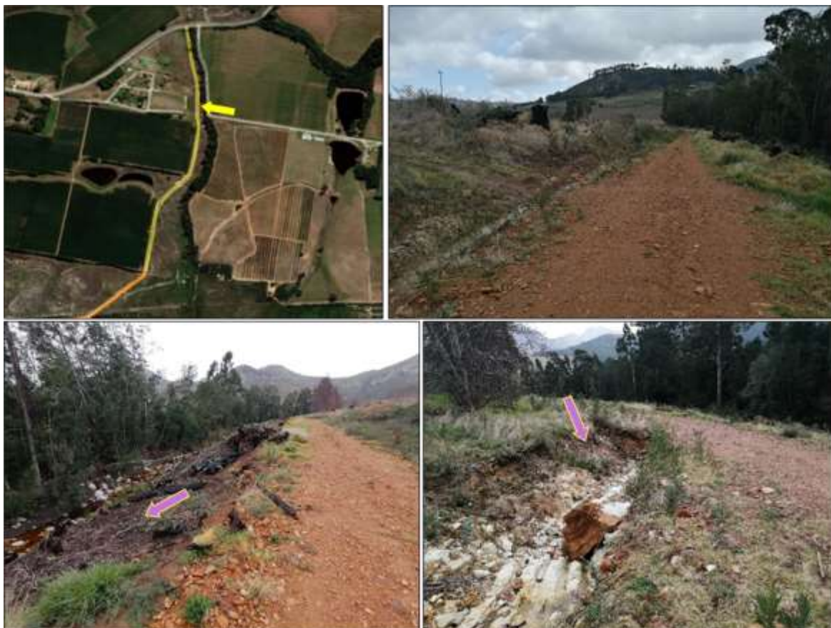
Figure 12: The northern section of the gravel road connecting to the tarred road on Portion 0 of Farm 296 (yellow line and arrow). This section displays fewer signs of erosion. It is however evident that some erosion has occurred in areas where alien vegetation has been removed, as well as in the stormwater furrows next to the road (pink arrows).
