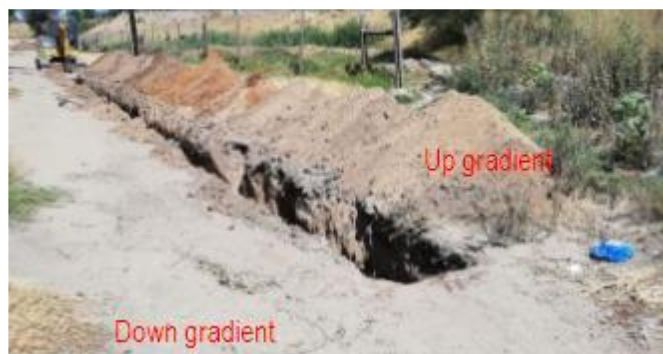
Figure 53: An example of a trench being excavated, and the removed soil stockpiled along the upgradient slope of the trench.
