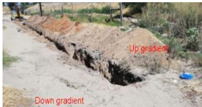
Figure 51: An example of a trench being excavated, and the removed soil stockpiled along the upgradient slope of the trench.
