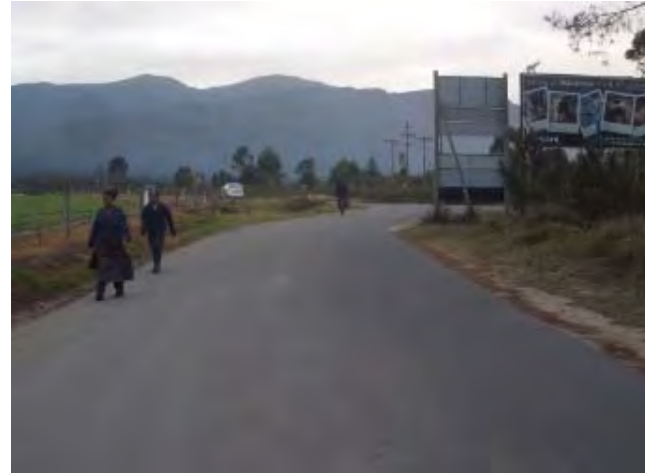
Photo 14: Northbound View along Mill Road approaching OP772
