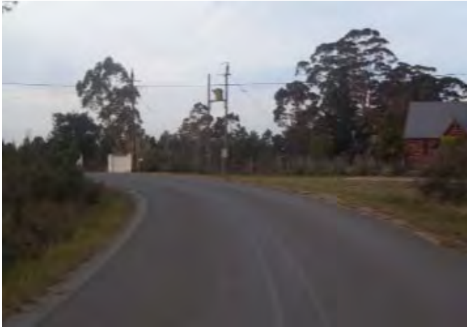
Photo 17: Southbound View along OP772 at sharp horizontal curve.
