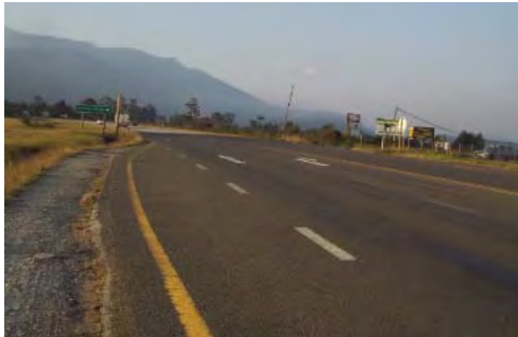
Photo 3: Northbound approach along N2 approaching OP772
