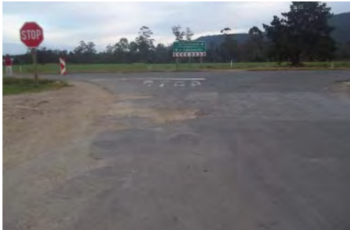
Photo 31: Westbound View along OP772 approaching the N2
