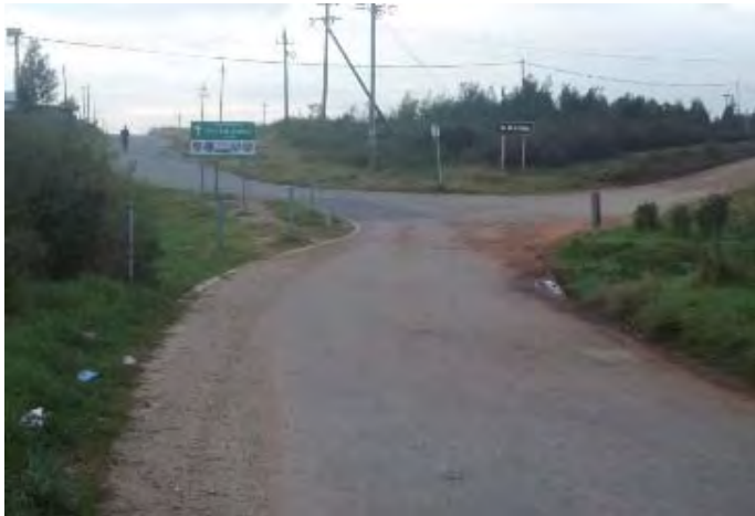
Photo 27: Eastbound view at OP772 / Wastewater Works Access Road intersection
