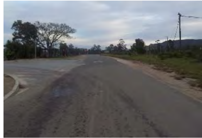
Photo 30: Westbound View along OP772 at Engen Filling Station Access
