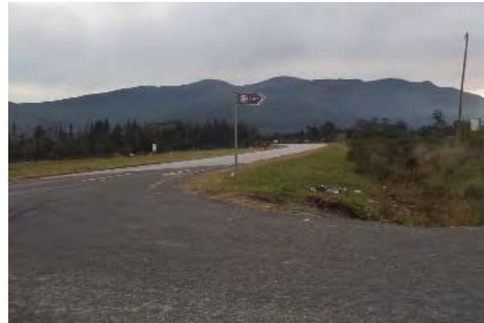
Photo 32: Shoulder sight distance to the north along the N2 from OP772
