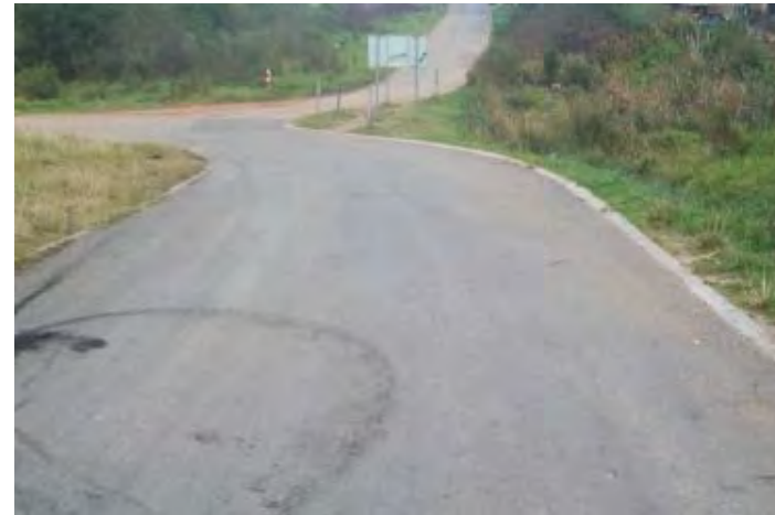
Photo 28: Westbound View along Wastewater Works Access Road toward OP772
