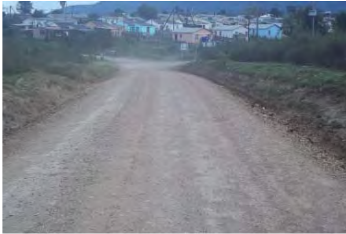
Photo 29: Northbound View along OP772 toward Wastewater Works Access Road
