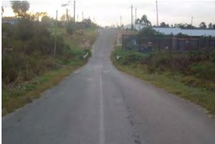
Photo 21: Eastbound View along OP772 east of Zimri Street
