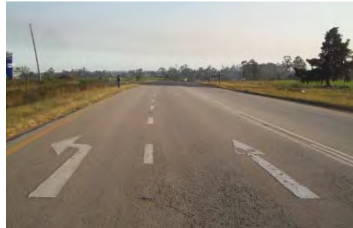
Photo 4: Southbound approach along N2 approach OP772
