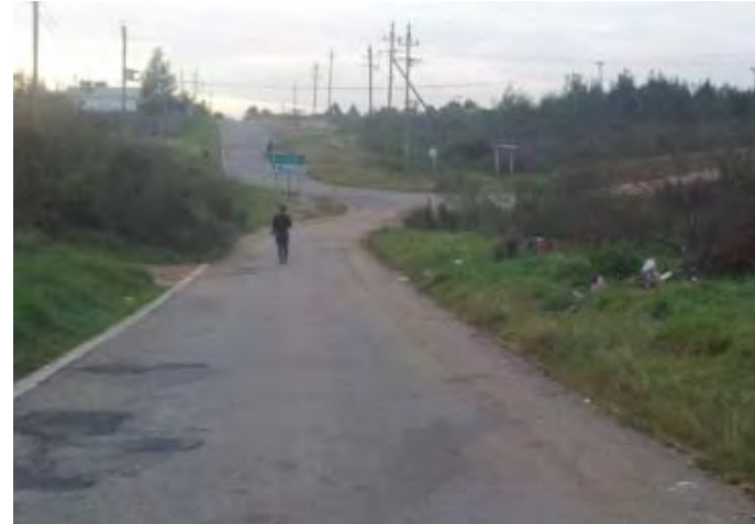
Photo 26: Eastbound View along OP772 approaching Wastewater Works Access Road
