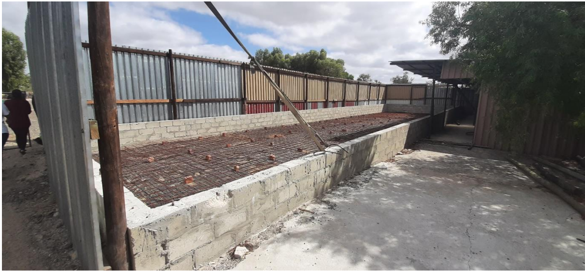
Figure 4: Partially constructed bund in 2022 - no further construction has occurred.
