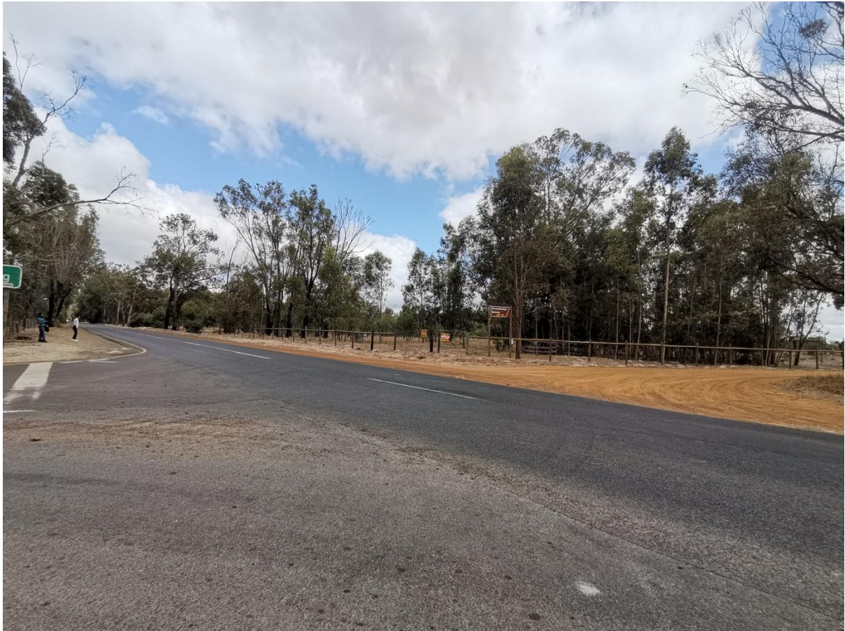
Figure 16: Access off of Klein Dassenberg Road onto Rondeberg Road (north-west facing).
