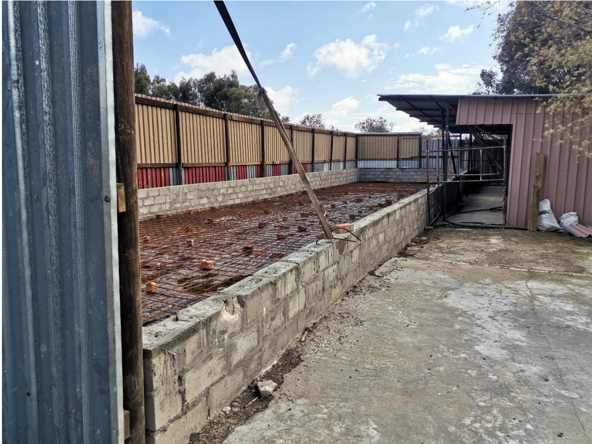
Figure 1: Transformation - bund partially constructed, 2021.
