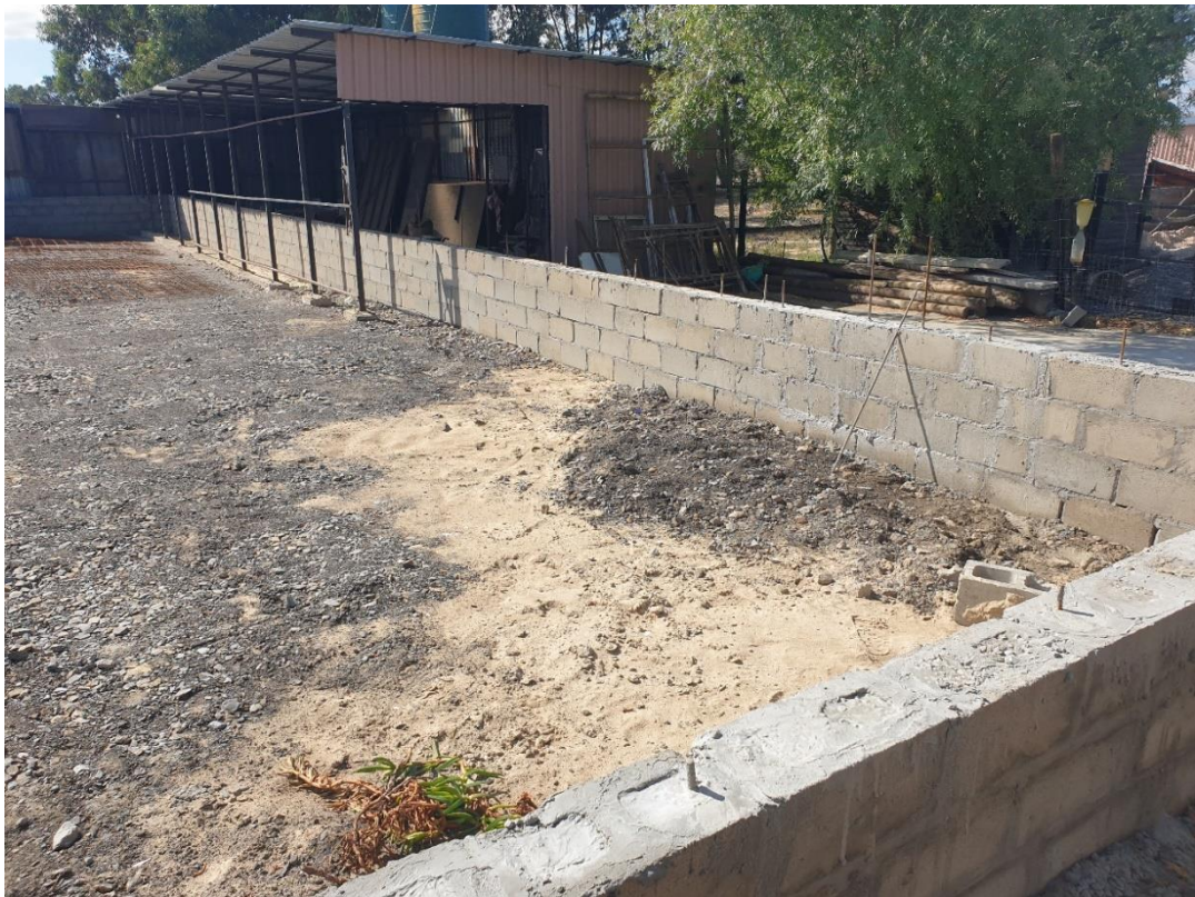
Photo 1: Commencement of the bund walls where tanks will be housed.
