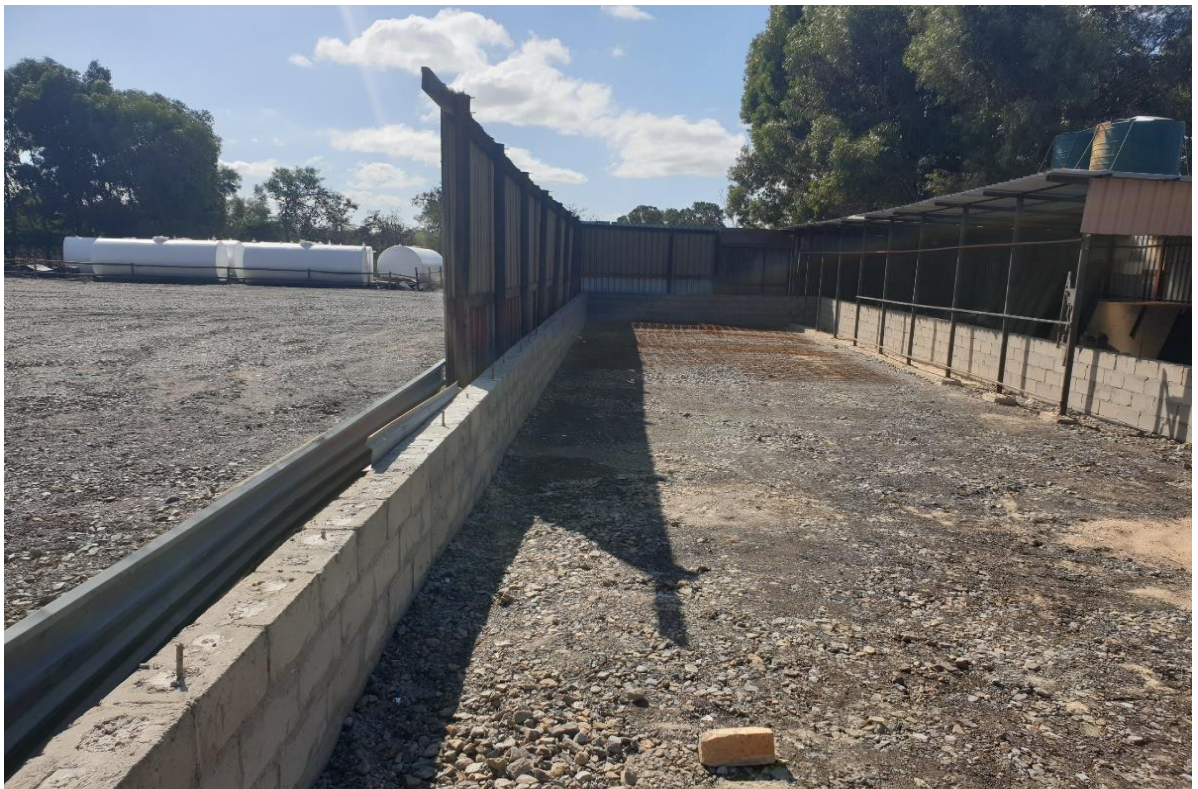
Photo 1: Commencement of the bund walls where tanks will be housed.
