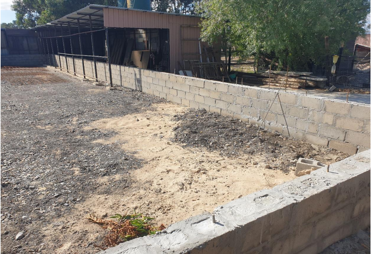
Photo 2: Commencement of bund walls.
