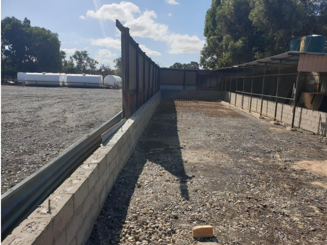
Photo 1: Commencement of the bund walls where tanks will be housed.
