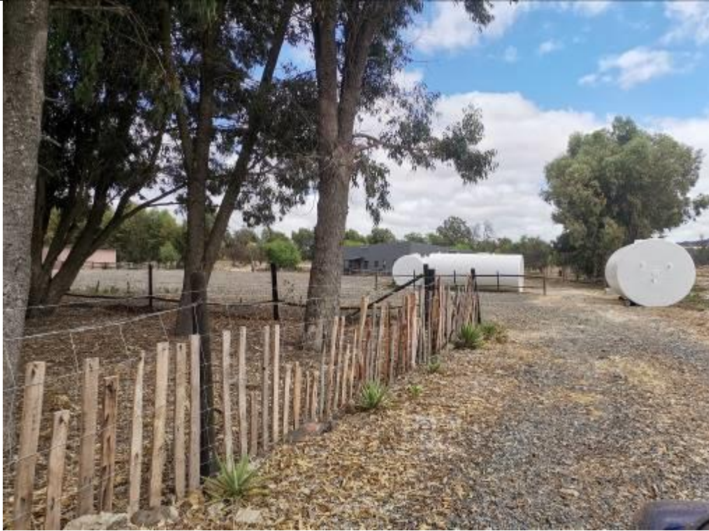
Figure 9: Gravelled preferred access (northern access) to turning area
