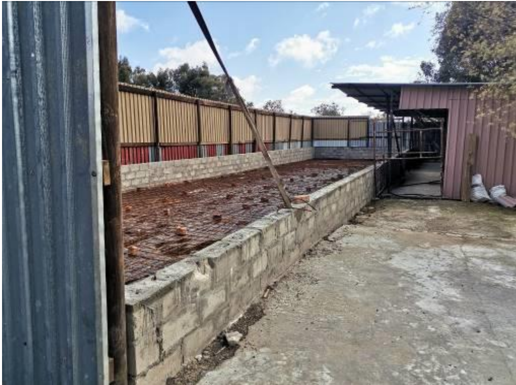
Figure 8: Bunded above-ground structure – incomplete
