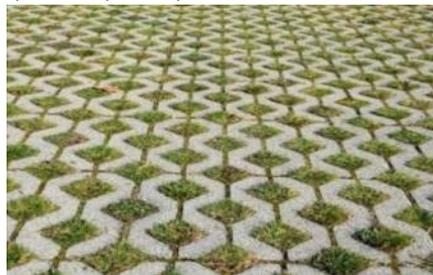
**Figure 17. An illustration of open pavers that can be incorporated into the design of this project for staff parking areas. This is not appropriate for truck parking areas on the site.**
