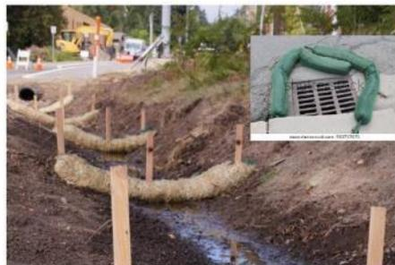
**Figure 20. Examples of silt socks placed perpendicular to the flow of water. These reduce the force of water flow, erosion, and can prevent unwanted sedimentation on the site.**
