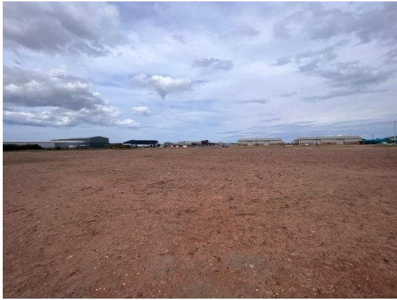
Figure 5. Site conditions upon initial site visit conducted by the EAP (October 2022).
