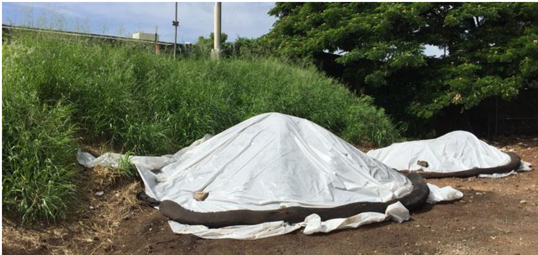
Figure 18: An example of a protected stockpile (imagfrom stormwaterhawaii.com).
