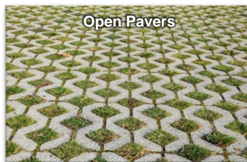
Figure 16: An illustration of open pavers that can be incorporated into the design of this project for staff parking areas. This is not appropriate for truck parking areas on the site.
