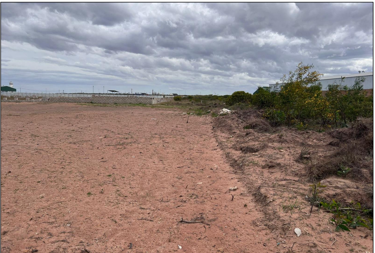
Looking north soon after grubbing.
