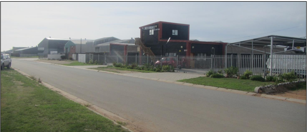
Neighbouring development across the road to the southeast.
