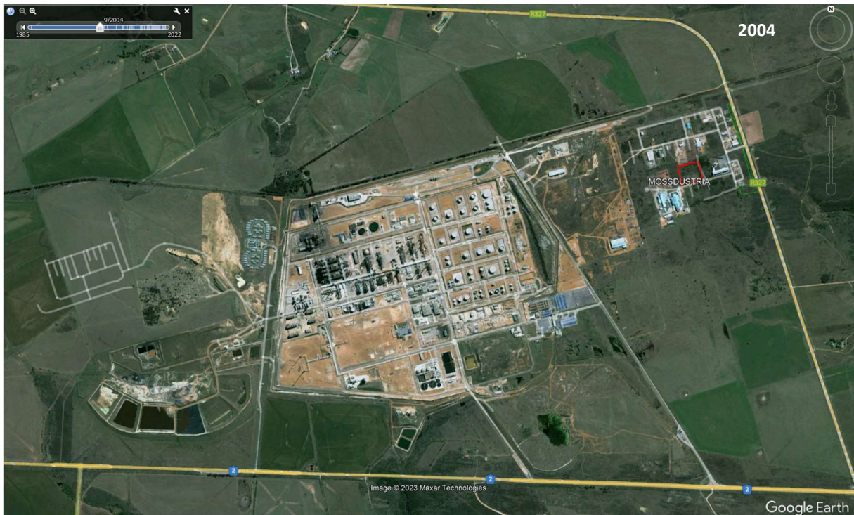
Historical satellite imagery from 2004 showing the site (red polygon) within the Mossdustria precinct
