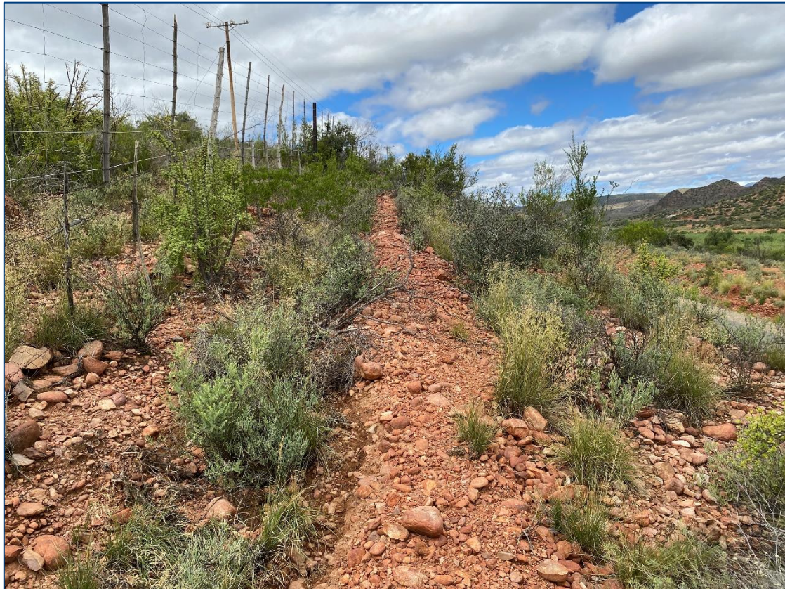
Figure 5-11: Partly vegetated slope above embankment with stormwater cut-off trench (WP8).
