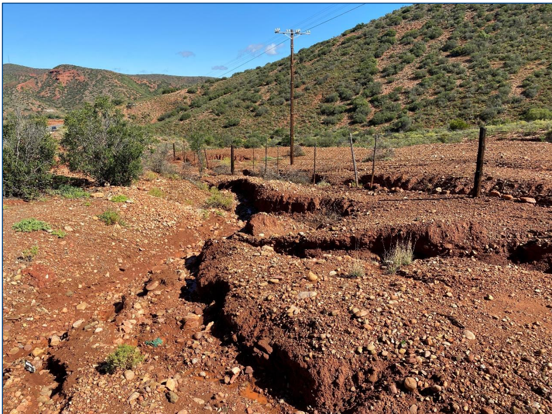
Figure 5-14: Eroded slope above road between WP12 and WP13.
