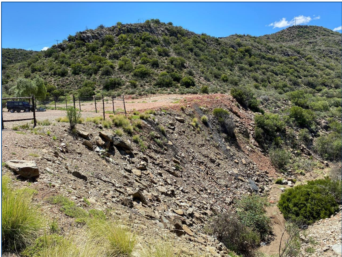
Figure 5-16: Excessive infilling at a lay-by, partly inside a watercourse (WP21).
