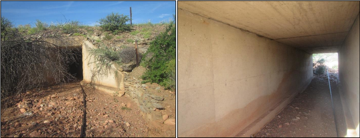
Figures 31 & 32: Two views of the culvert at waypoint 728.
