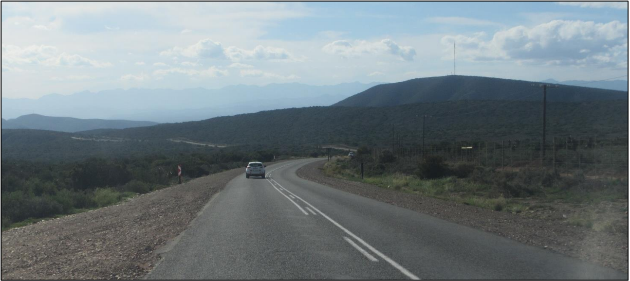
Figure 22: View northbound at the southern end of the study area.
