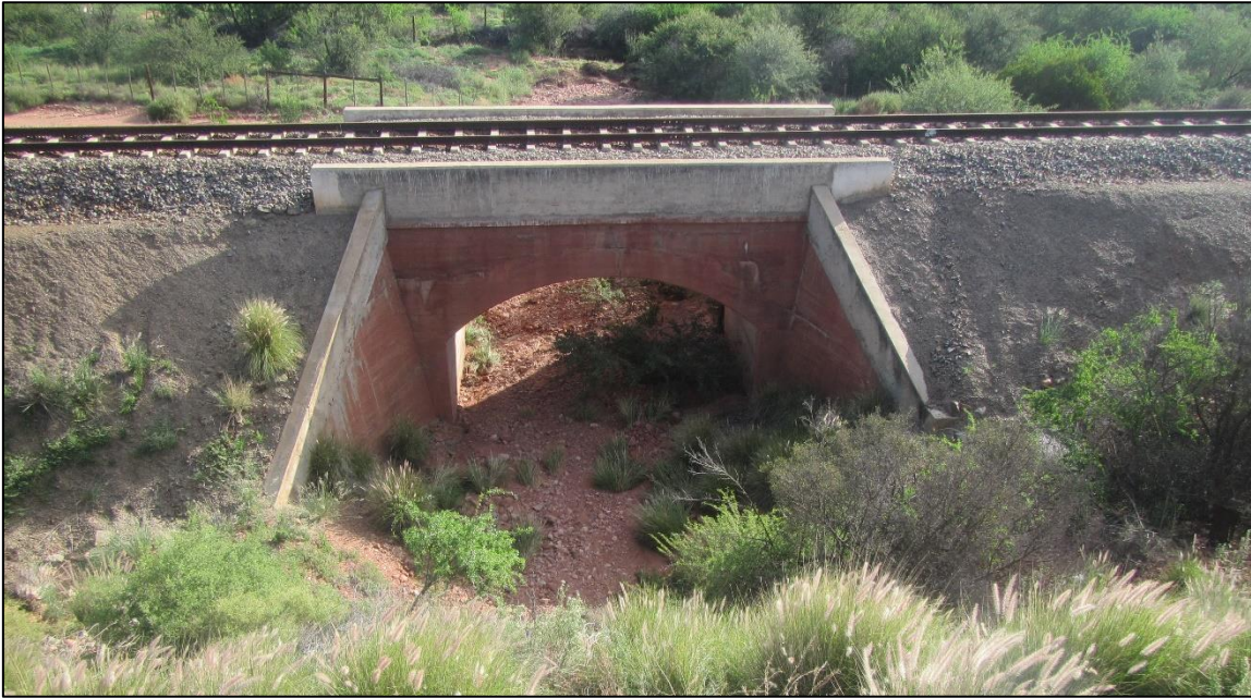
Figure 35: Railway culvert at waypoint 730.
