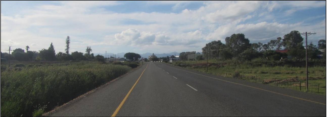
Figure 8: Looking north near the southern edge of Oudtshoorn.
