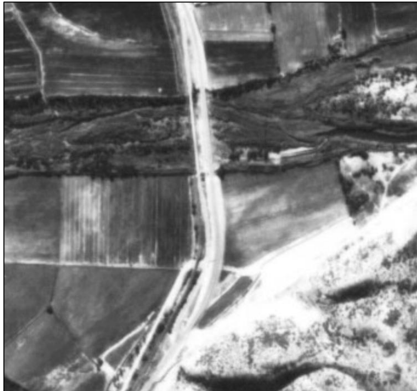
Figure 42: 1979 aerial view showing the modern bridge in place immediately east of the old one.
