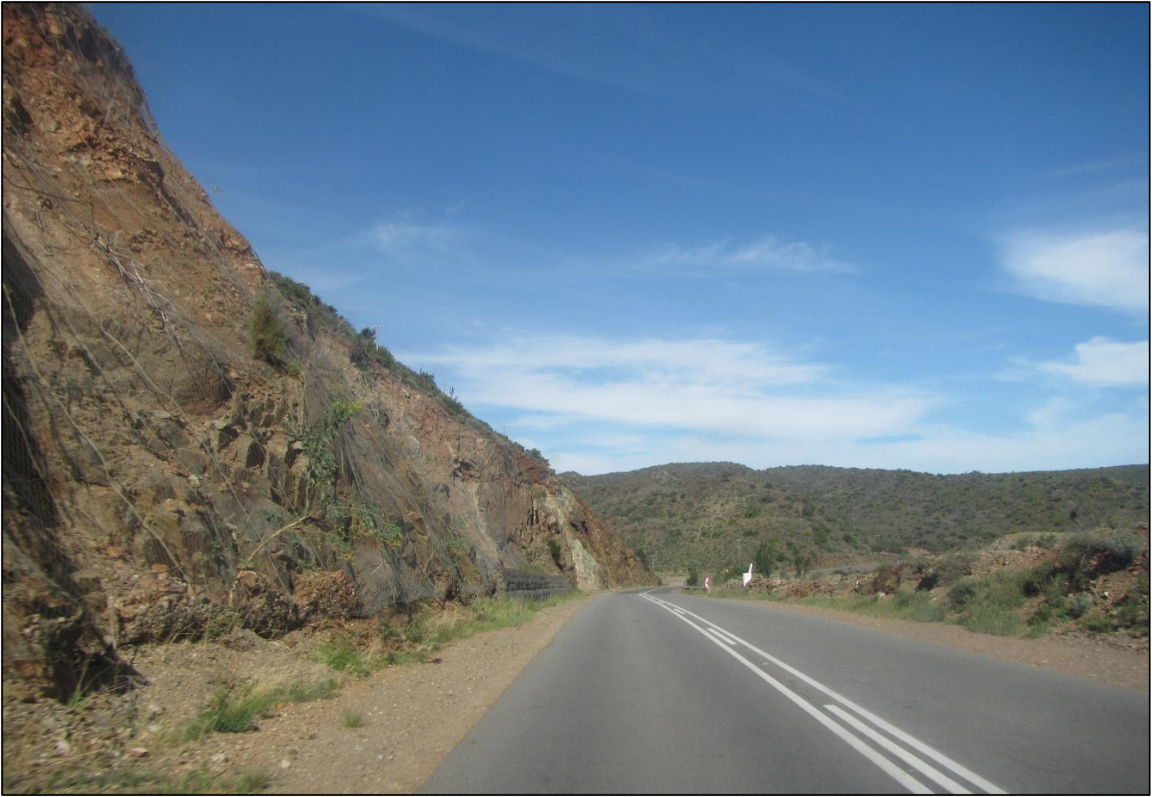
Figure 16: View southbound showing a tall road cutting stabilised with metal mesh.
