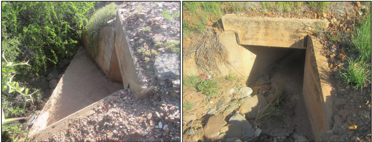
Figures 27 & 28: Two views of the culvert at waypoint 725.
