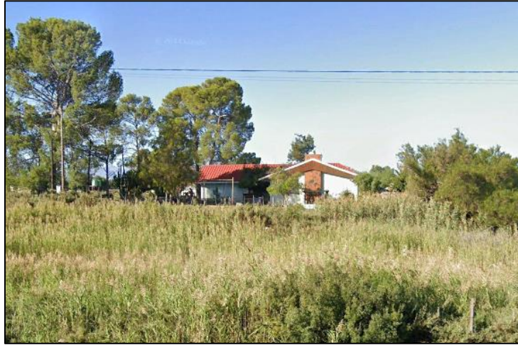
Figure 44: The house located 65 m east of the N12.
