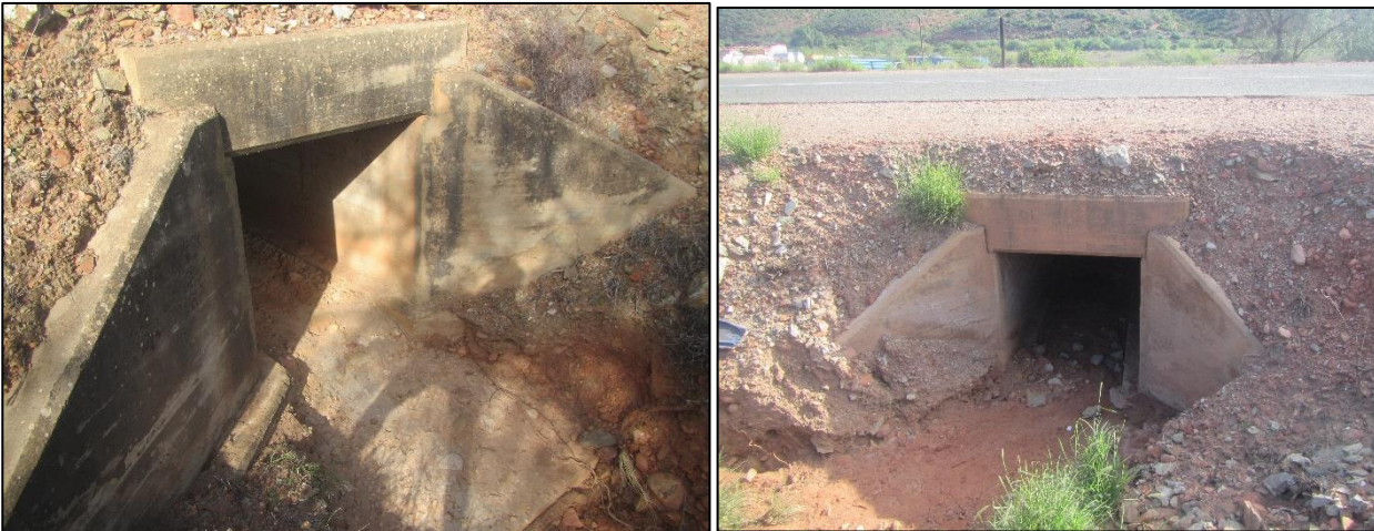
Figures 33 & 34: Two views of the culvert at waypoint 729.
