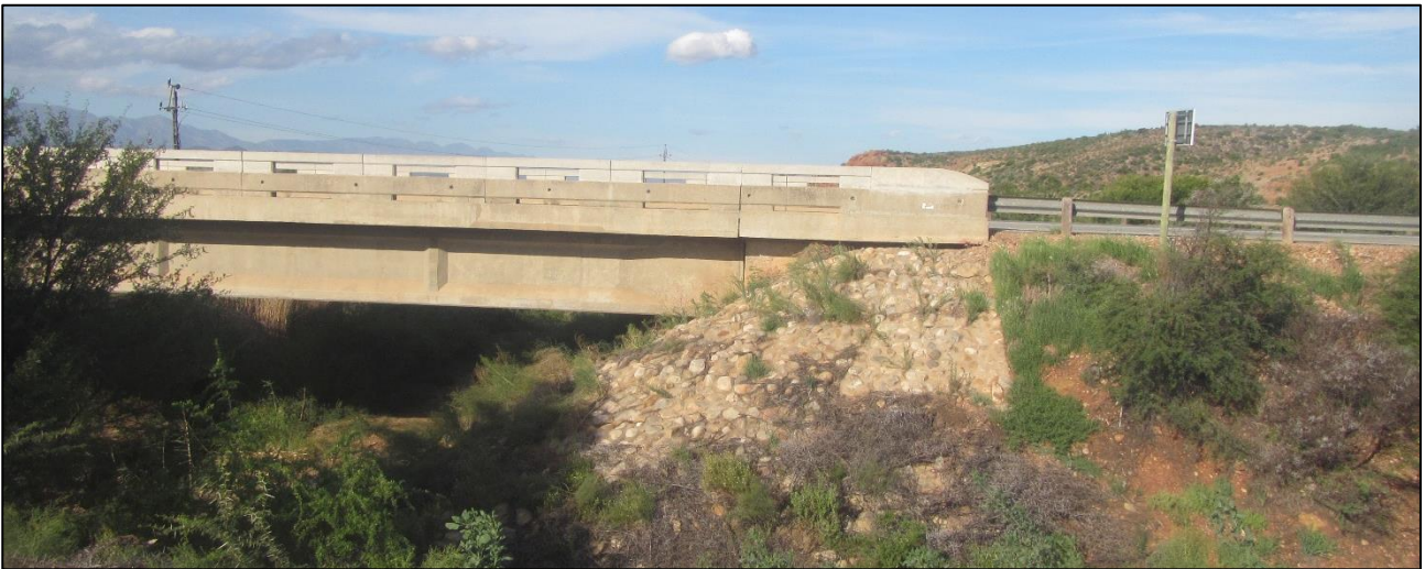
Figure 38: The current N12 road bridge.
