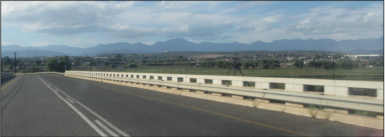
Figure 37: View along the modern N12 bridge.
