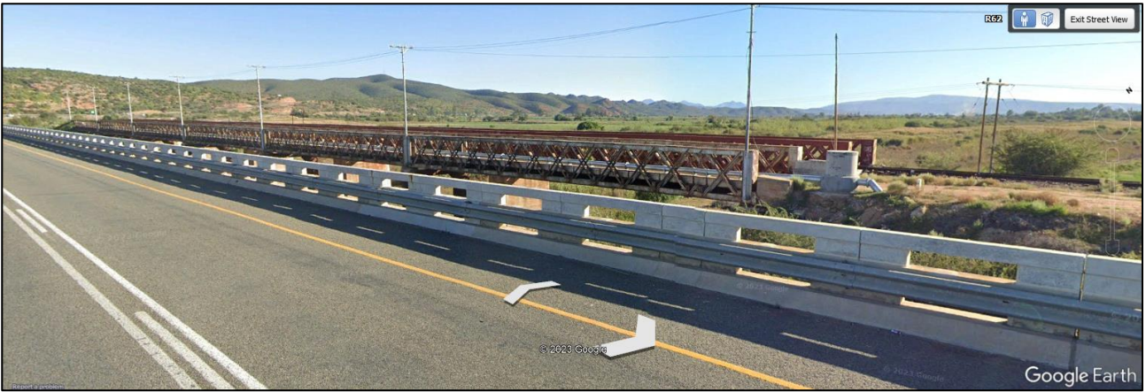
Figure 40: View from the N12 towards the old road bridge (now carrying a pipeline) and the railway bridge in the background.
