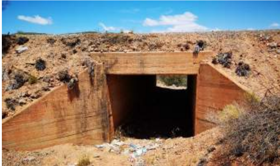
Photo 10.2 TYPICAL MAJOR CULVERT ALONG THE ROUTE
