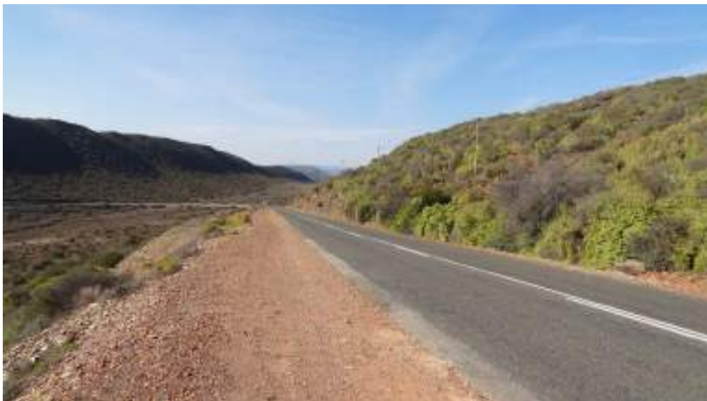
Photo 4.1 TYPICAL CROSS SECTION (km 19.40) LOOKING TOWARDS OUDTSHOORN
