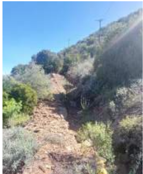
Close-up of cut-off drain.
