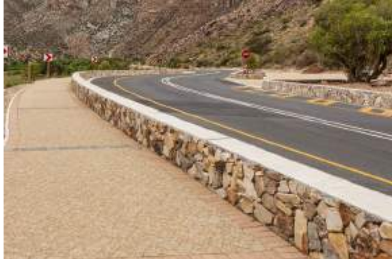
Photo 17.1 EXAMPLE OF STONE MASONRY WALL ON TR31/2 IN COGMANSKLOOF
