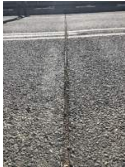
Joint condition at visual inspection conducted 2019.
