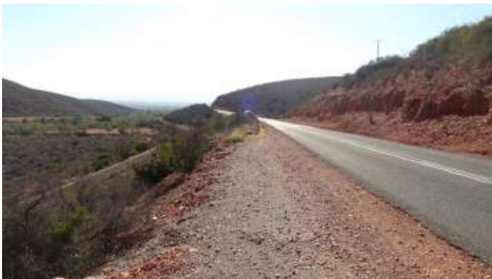
Photo 4.3 TYPICAL CROSS SECTION (km 24.90) LOOKING TOWARDS OUDTSHOORN
