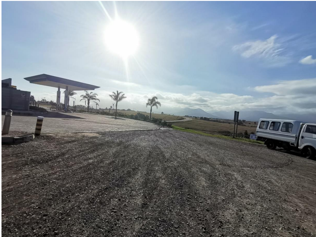
Figure 10: Existing Sasol garage meets Portion 278, access to be utilized and maintained via the Sasol Garage.
