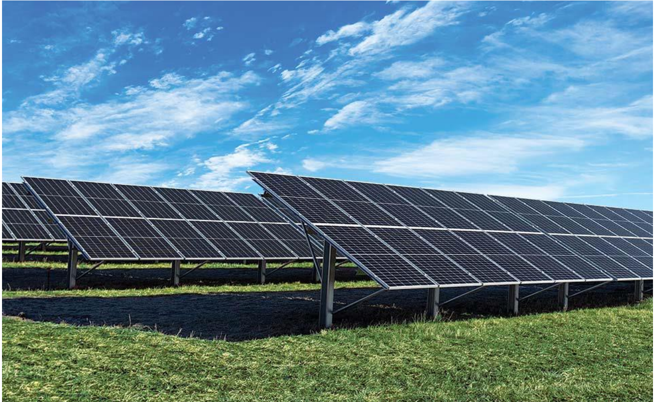
Figure 9: Typical Fixed-tilt Ground-mount System (2V Arrangement)
