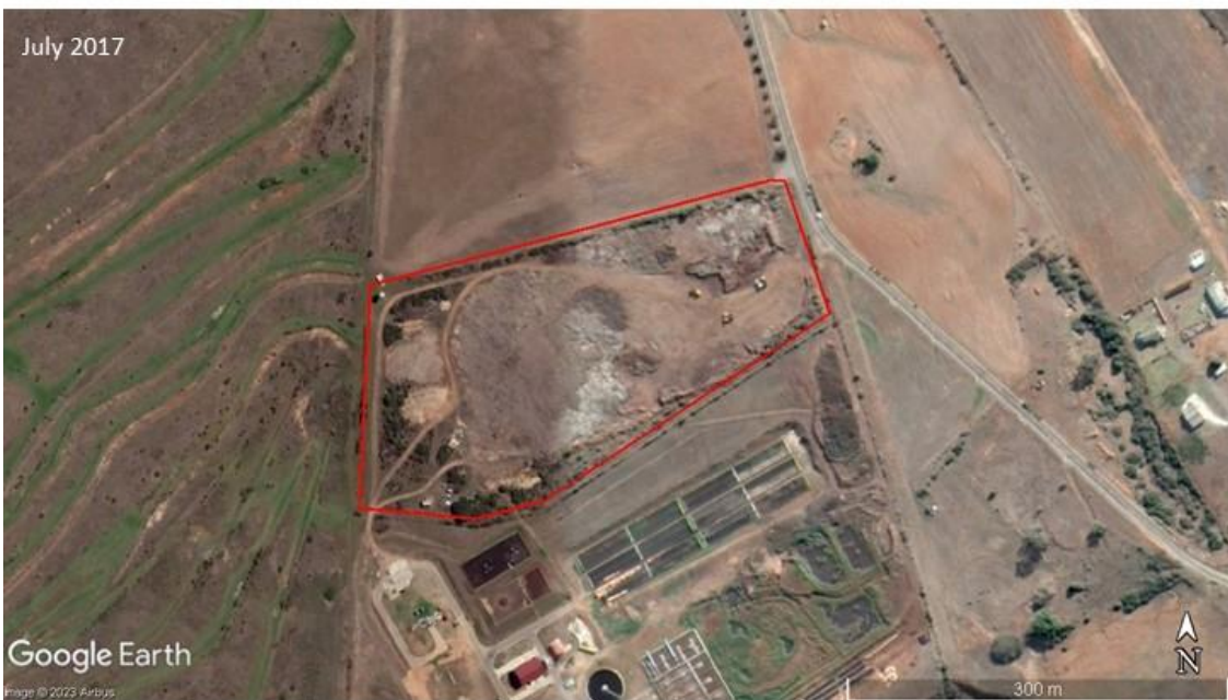
Figure 39: Further evidence of dumping and spreading of stockpiles in 2016 and 2017. Courtesy of Google Earth 2023. (Source: Heritage Statement in support of Heritage Western Cape Notification of Intent to Develop (HWC NID – Section 38), Proposed Hartenbos WWTW PV Solar Plant on a Portion of RE/101/217 of Farm Hartenbosch, Mossel Bay Municipality, Western Cape Province, 2023, Prepared by Dr. Peter Nilssen)(Appendix G4).
