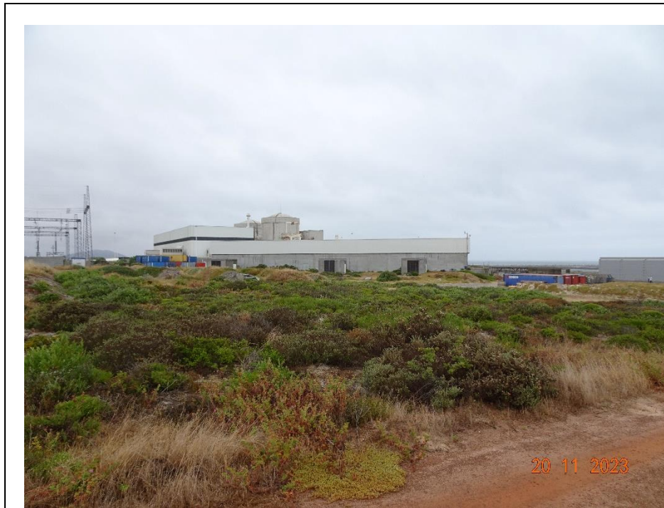
Figure 1 – View of the proposed development site from the Northern access road.
