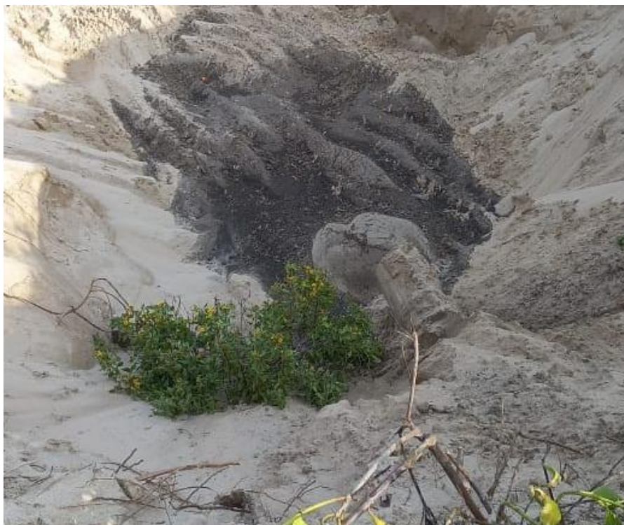
Figure 10: Pipe outlet of sump 1.
