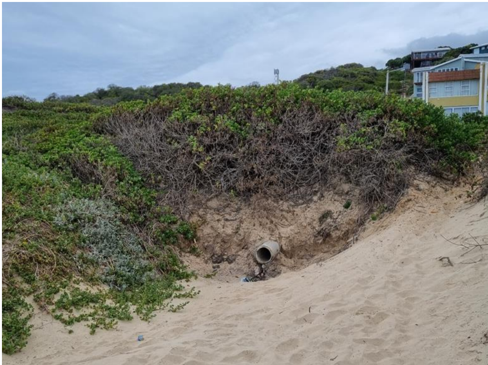
Figure 12: Pipe outlet of sump 2.
