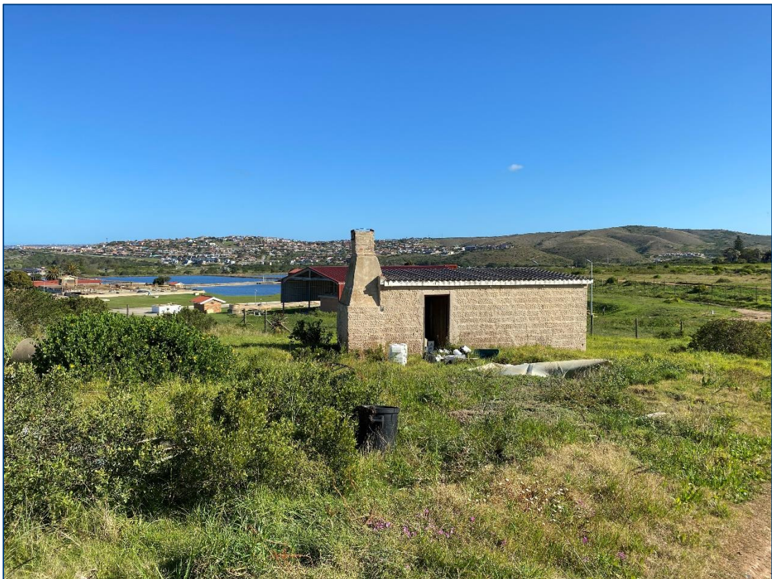
Figure 5-6: Abandoned dwelling in the south-western corner of the site.
