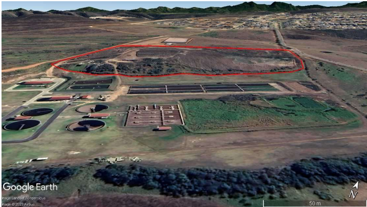
Figure 10. Oblique NNE view of the study area (red polygon) showing the raised “made ground” north of the Hartenbos WWTW. The residential development of Monte Christo is in the top right background. Courtesy of Google Earth 2023.
