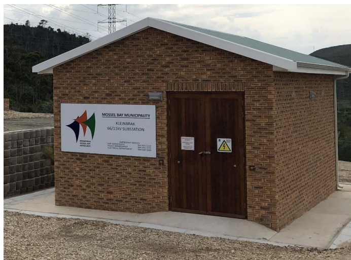
Figure 13: Typical Brick Built substation to house the MV switchgear.
