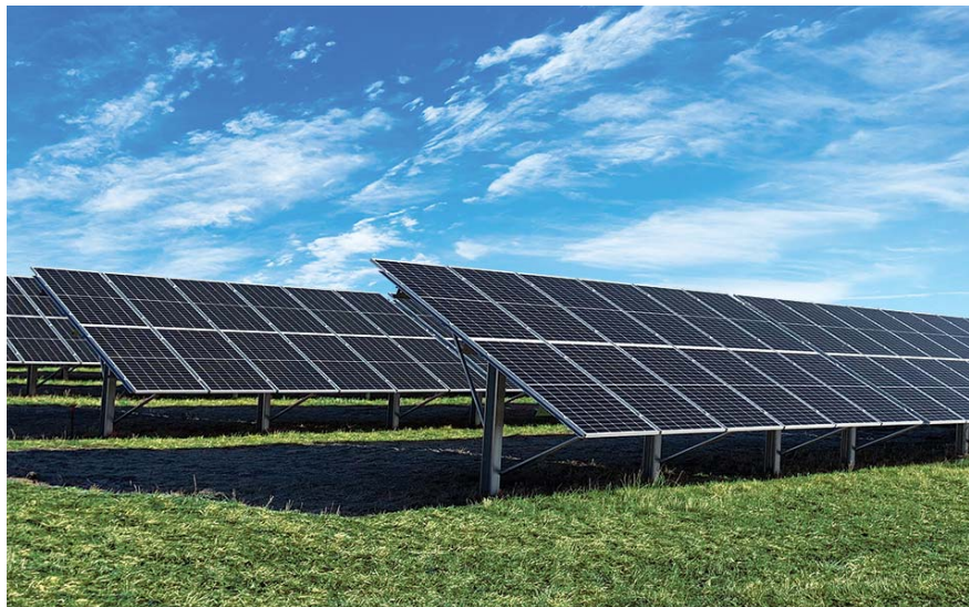
Figure 9: Typical Fixed-tilt Ground-mount System (Source: Element Consulting Engineers)
