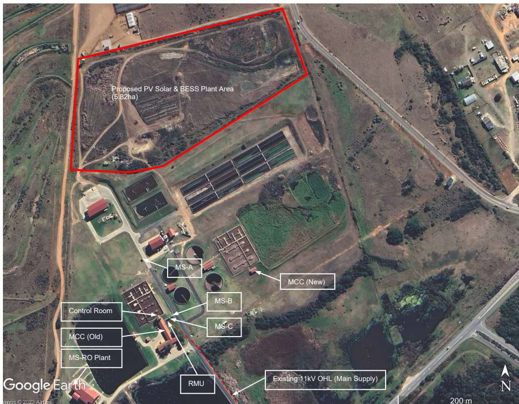
Figure 3: Location of the proposed PV Solar Plant site in the Hartenbos WWTW site (Source: Element Consulting Engineers)
