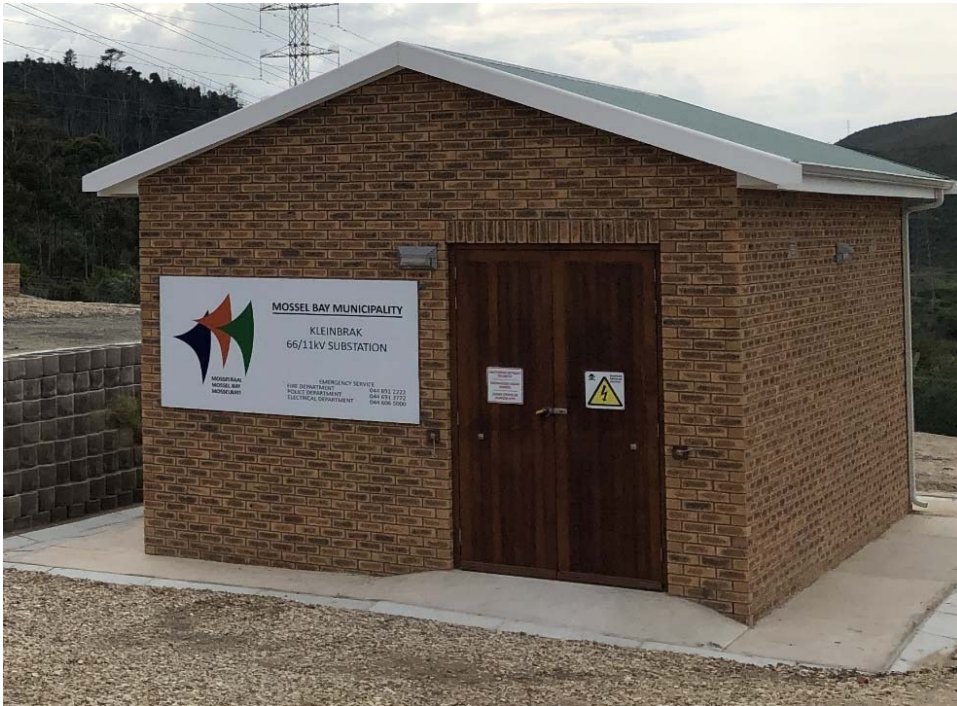
Figure 4-18: Typical MV Substation Building (External)
