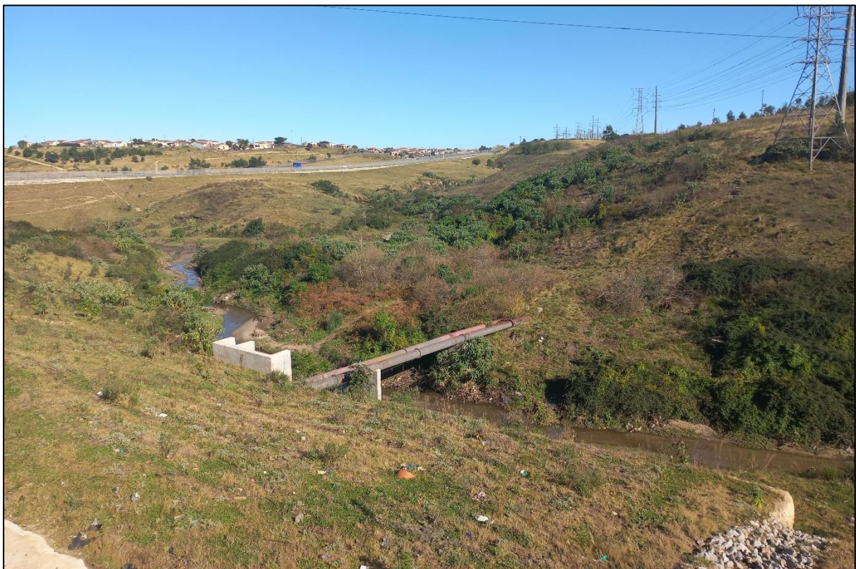
Plate 1: A photograph of the Skaapkop River at the rising main pipeline crossing.
