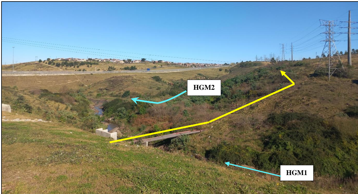
Plate 2: Photograph showing the approximate pipeline route requiring upgrades in yellow
