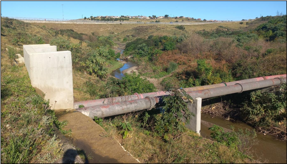
Plate 3: A photograph showing the Skaapkop River (HGMI) crossed by an existing pipeline on site
